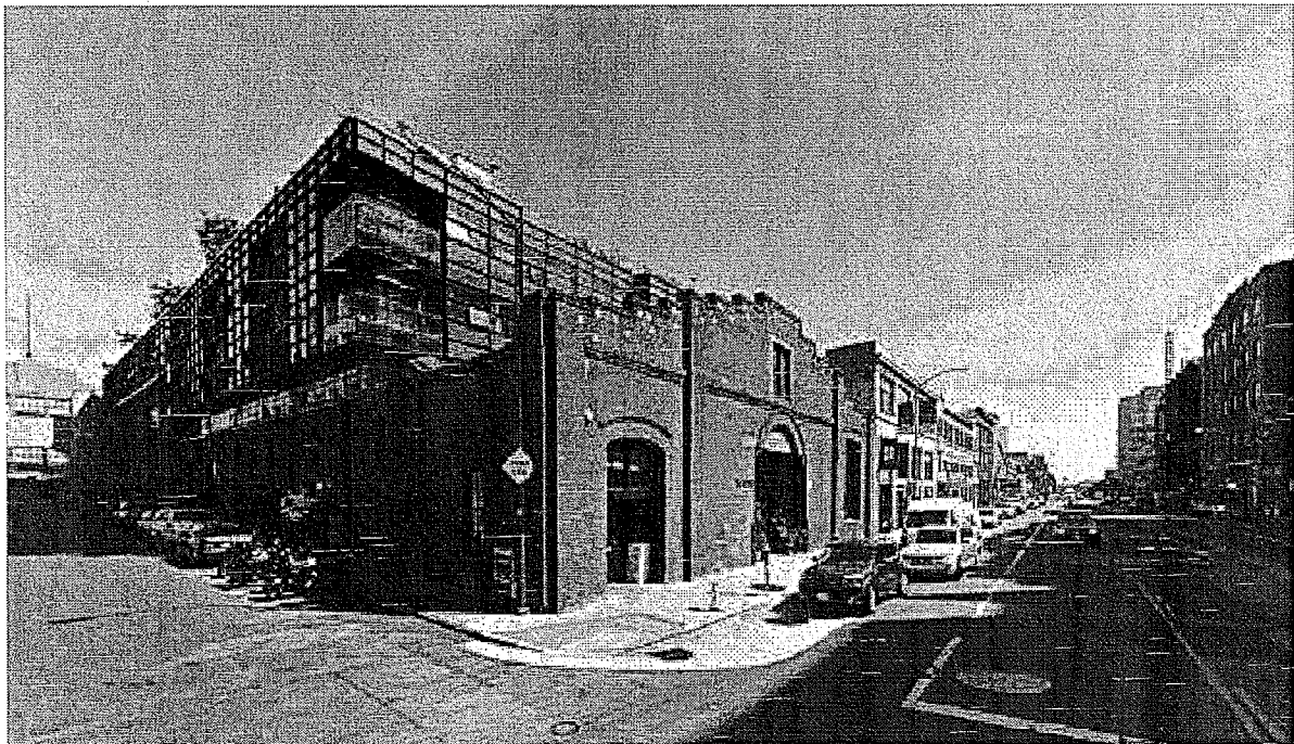
FIGURE 2.7 166-178 Townsend St (2016, After Construction)
