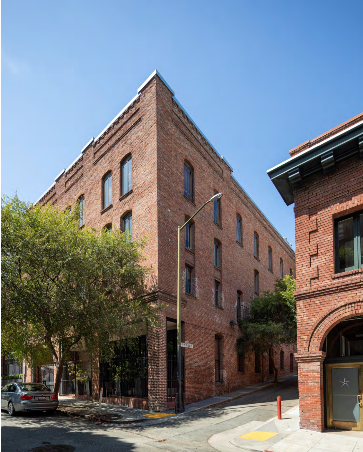
View looking northwest at corner of Pacific Avenue and Osgood Place, showing primary (south) and east façades (Henrik Kam, 2019).
