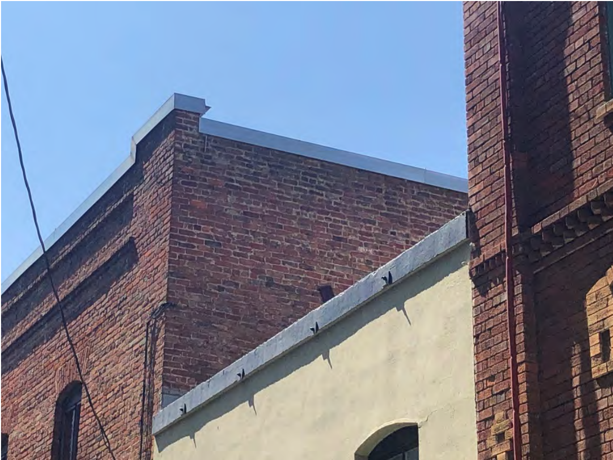
Figure 23: Partially visible north (rear) façade, 2020. Looking southwest.
