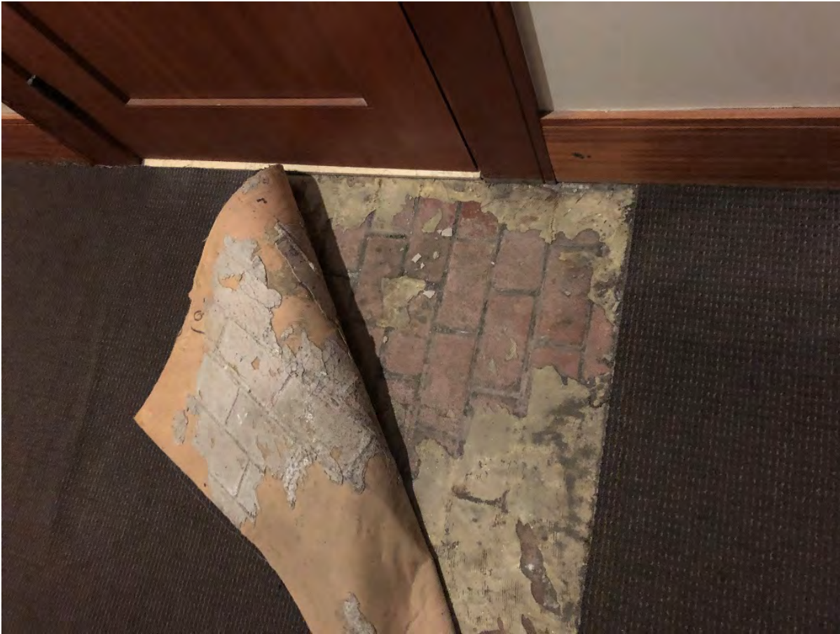
Figure 28: Detail of brick floor beneath the carpet at the ground floor, 2020. Further investigation is needed to determine if it is historic.
