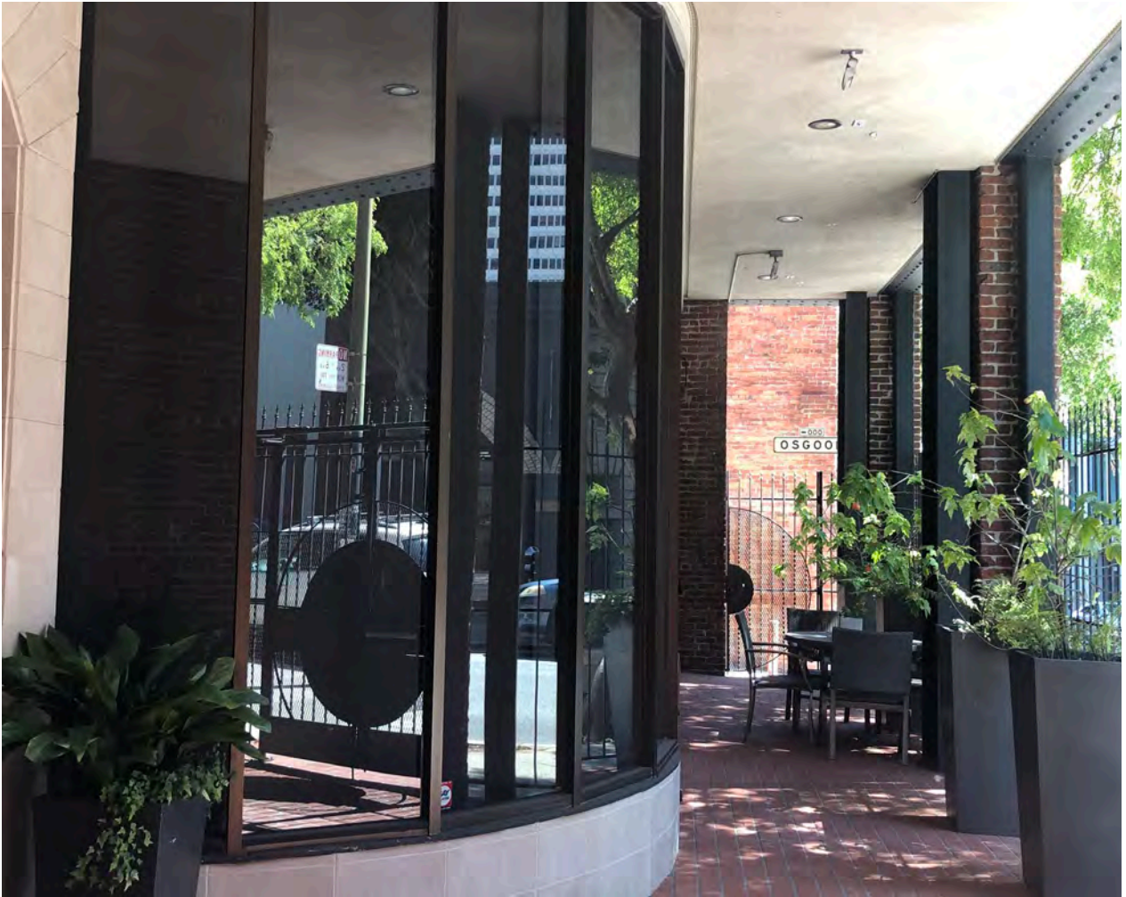
Figure 17: Storefronts within arcade along primary façade at Pacific Avenue, 2020. Looking east.
