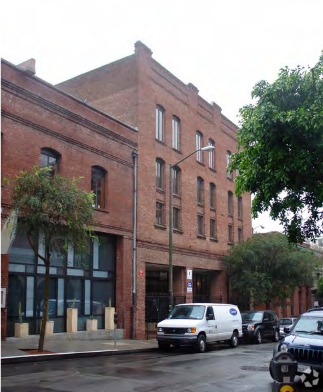
Figure 19: Primary façade at Pacific Avenue, 2019. Looking northeast. Courtesy of Henrik Kam
