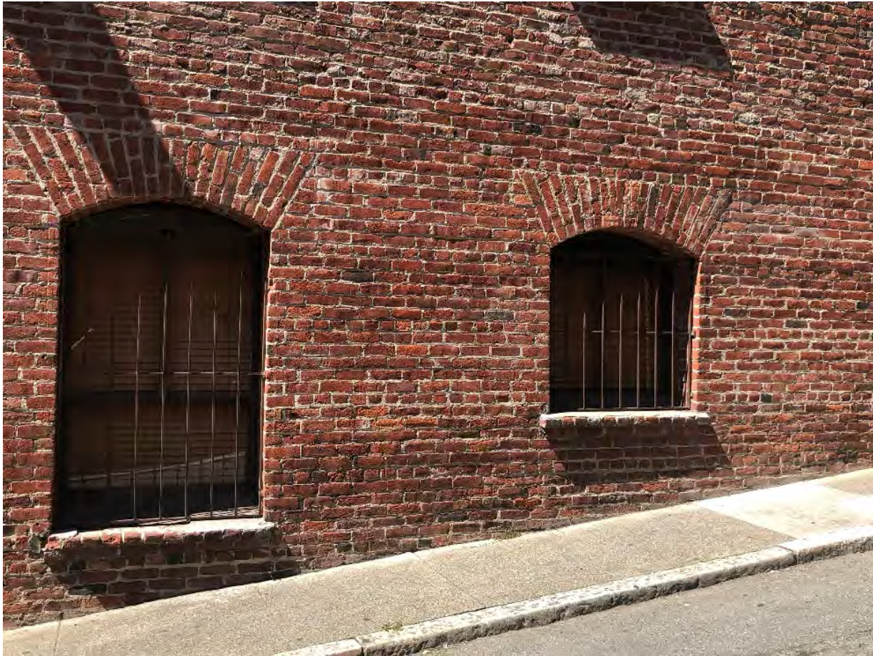
Figure 21: Grilles at windows at Osgood Place façade, 2020. Looking west.
