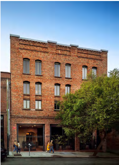
Figure 5: Primary façade, 2019. Looking north. Courtesy of Henrik Kam.
