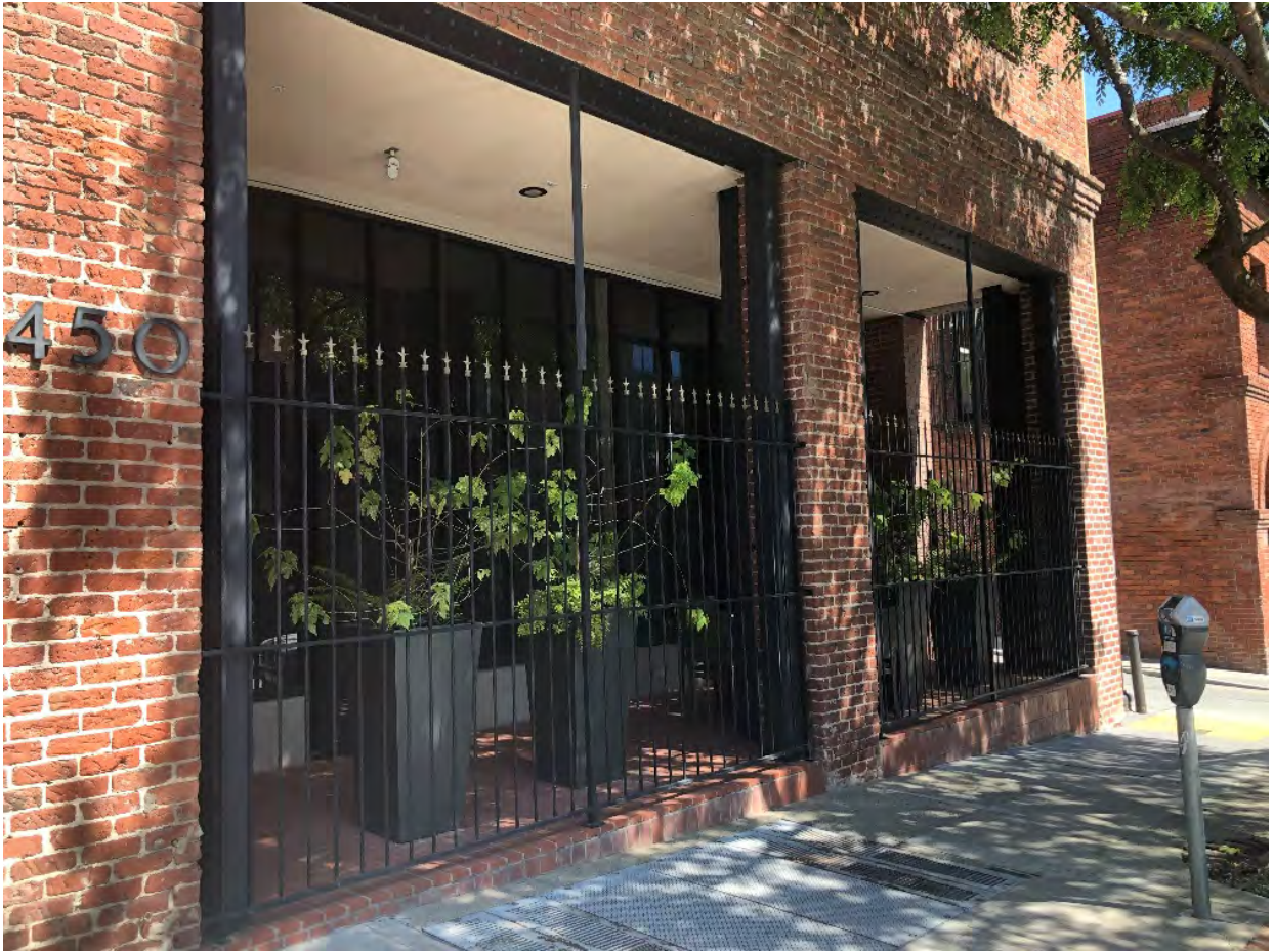
Figure 12: Storefronts at ground floor of primary façade, 2020. Looking northeast.
