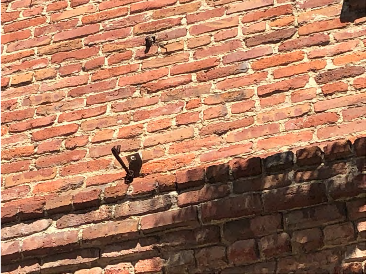
Figure 14: Simple brick cornice above storefronts at primary façade (Pacific Avenue), 2020. Looking north.
