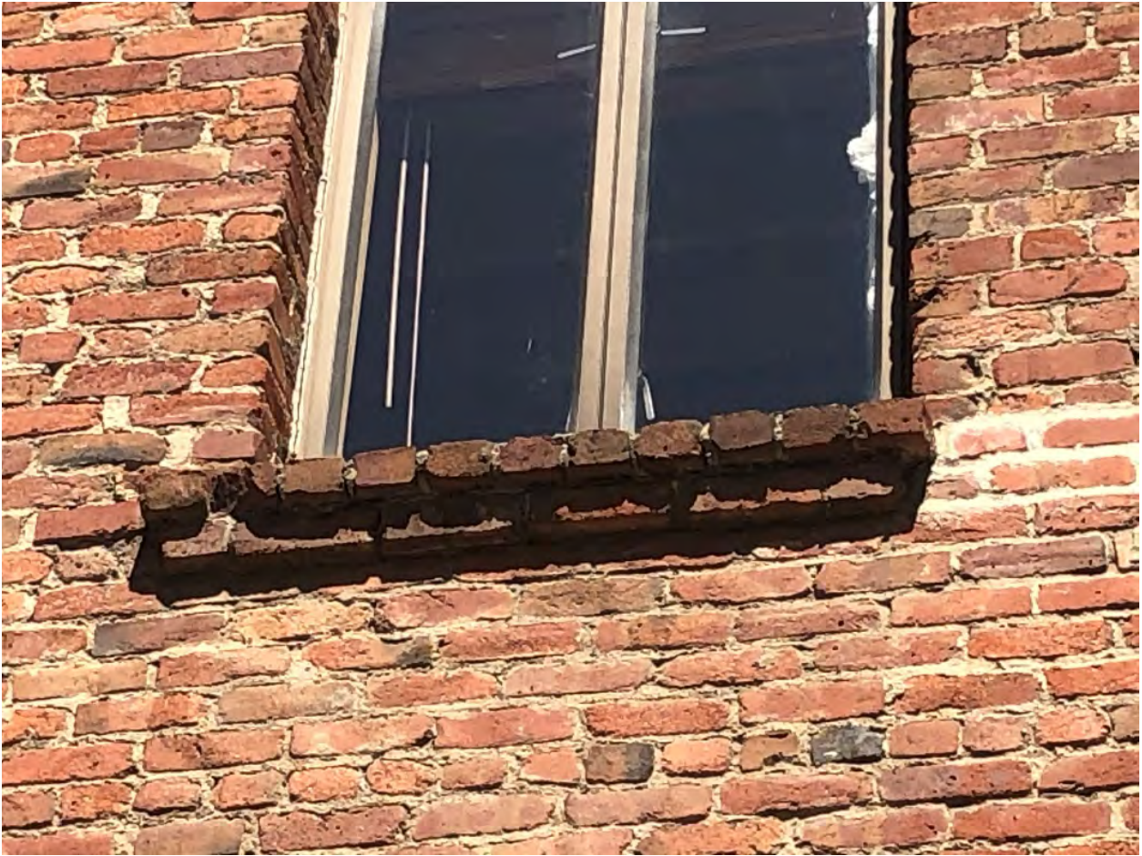
Figure 10: Brick sill detail at primary (Pacific Avenue) façade, looking north. 2020.
