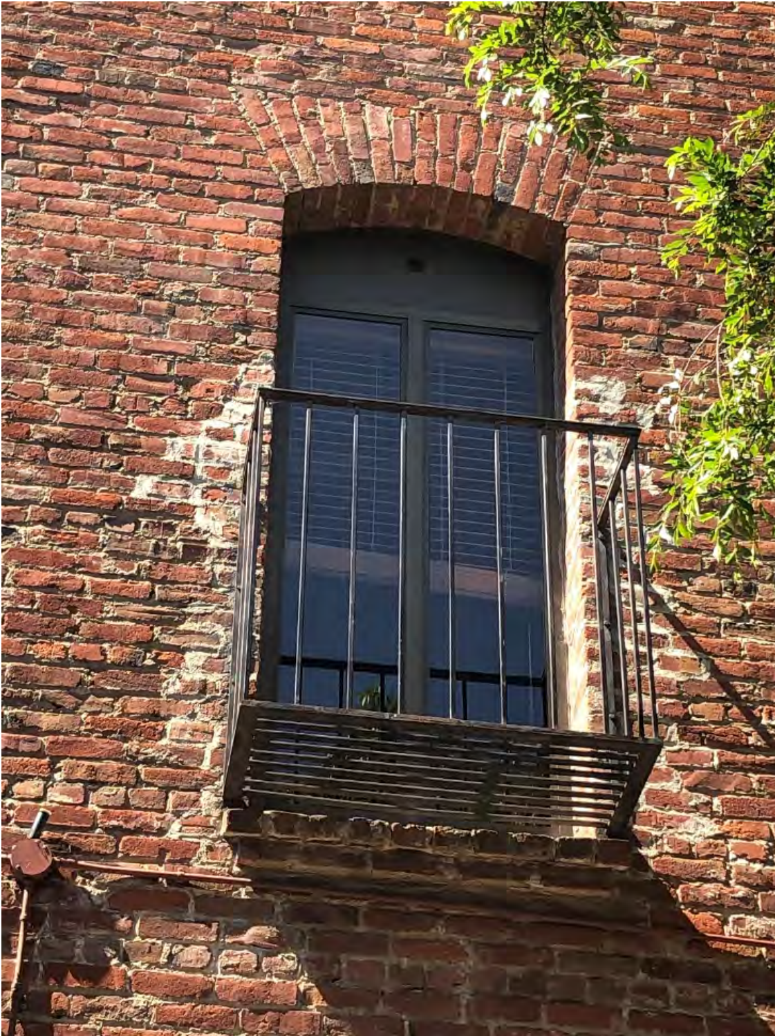
Figure 22: Balcony rail at Osgood Place façade, 2020. Looking west.
