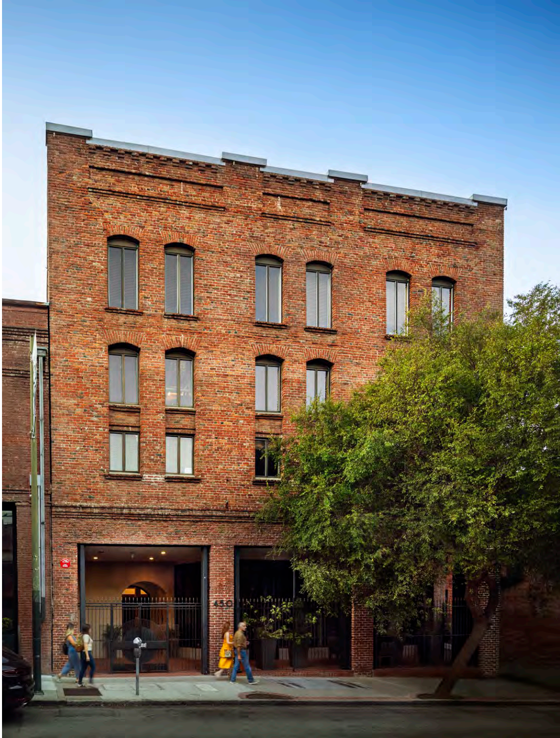
Pacific Avenue - South Elevation (Henrik Kam, 2019).
