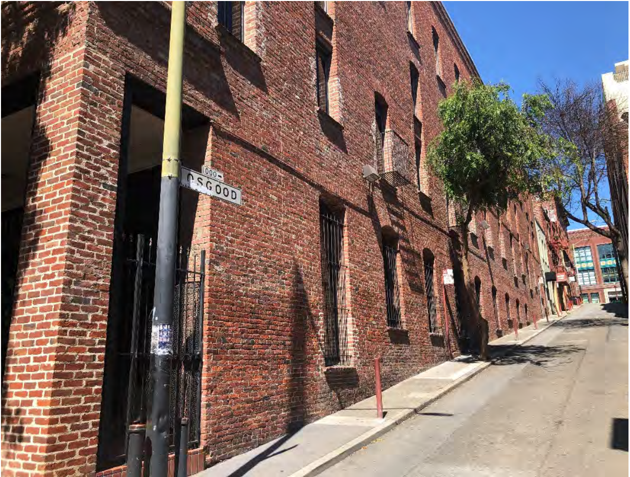
Figure 13: Ground floor along Osgood Place, 2020. Looking northwest.
