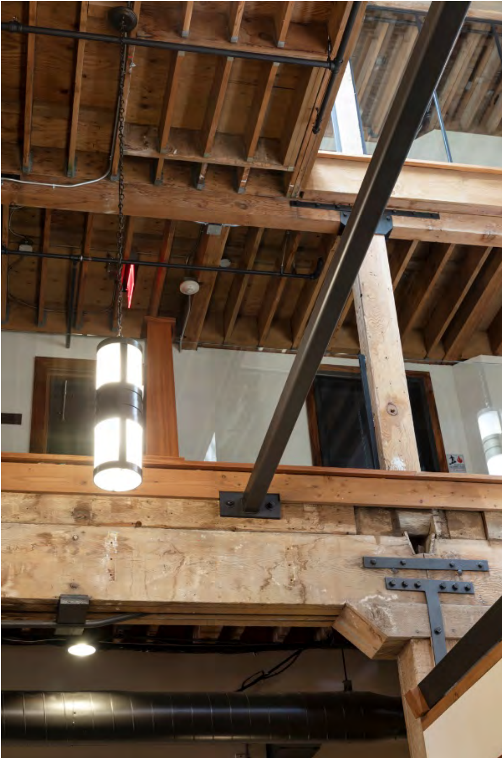
Figure 26: Wood support pillar from ground to third floor, 2019. Looking west. Courtesy of Henrik Kam.
