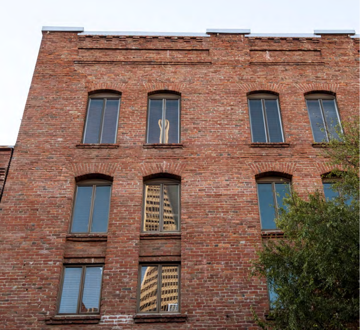
View looking up at south façade, Pacific Avenue (Henrik Kam, 2019).
