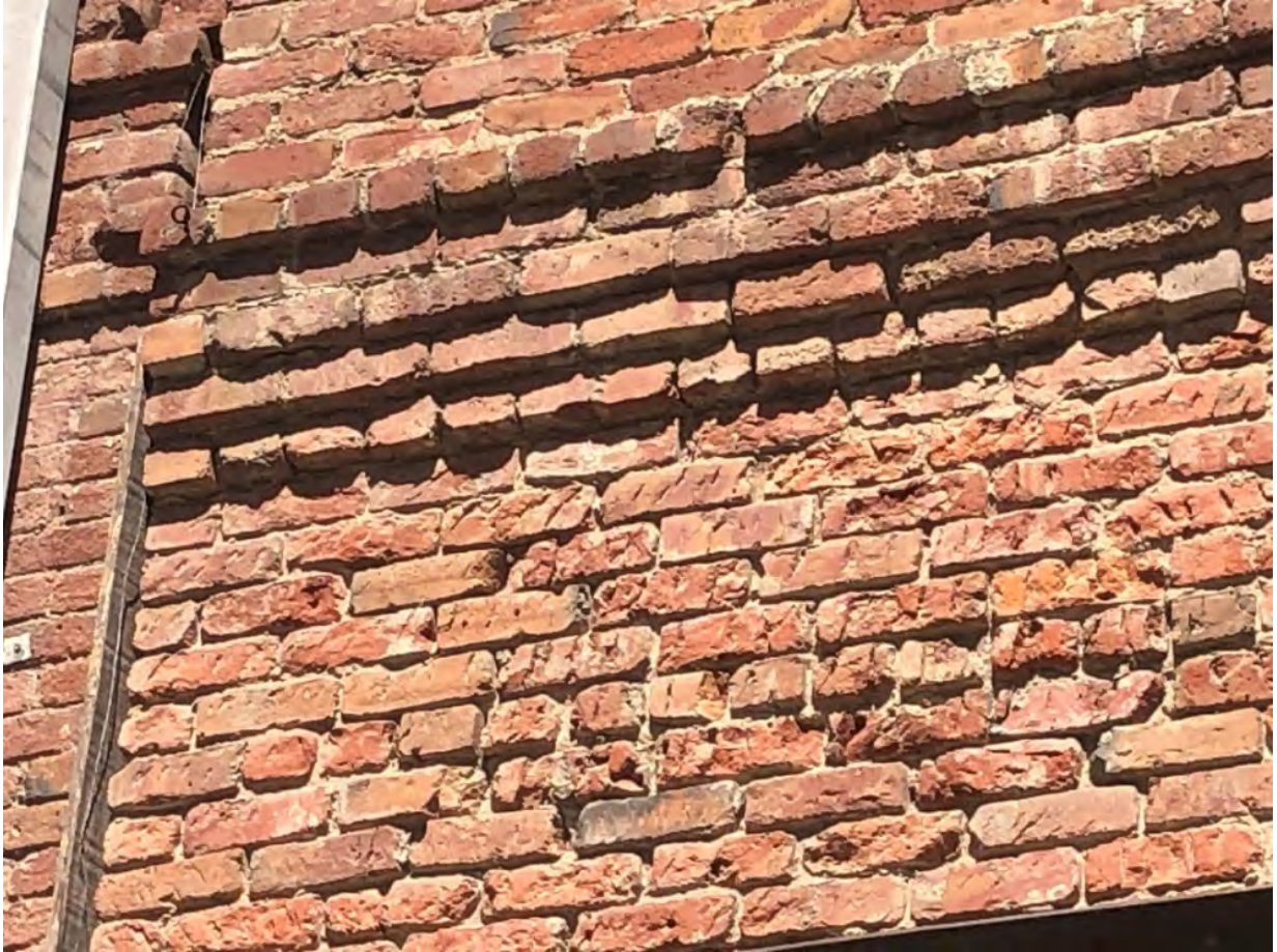
Figure 11: Simple brick cornice above storefronts at primary (Pacific Avenue) façade, looking north. 2020.
