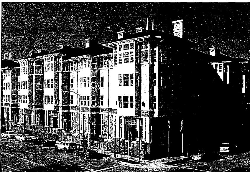
An example of strong vertical orientation, varied rooflines and massing breaks
