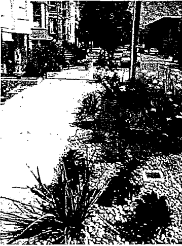
Permeable sidewalk features allow for stormwater to infiltrate
