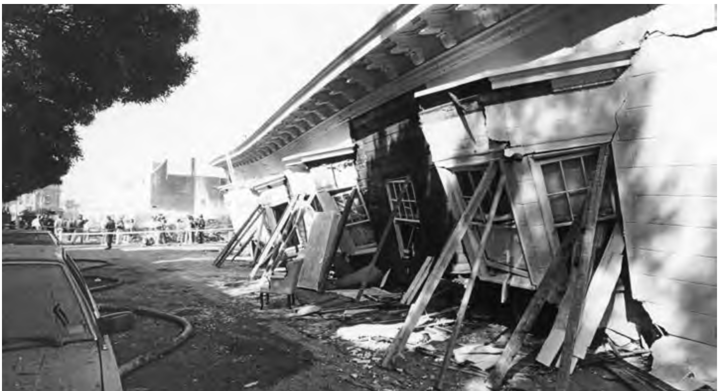
Aftermath of the 1989 Loma Prieta Earthquake
