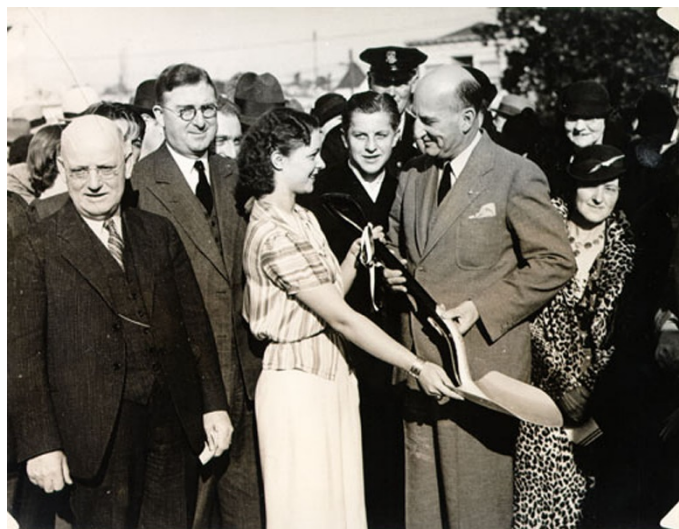
Figure 51. Groundbreaking for the Sunshine School, 1935. Source: San Francisco Historical Photograph Collection, San Francisco Public Library, Photo ID# AAD-4255
