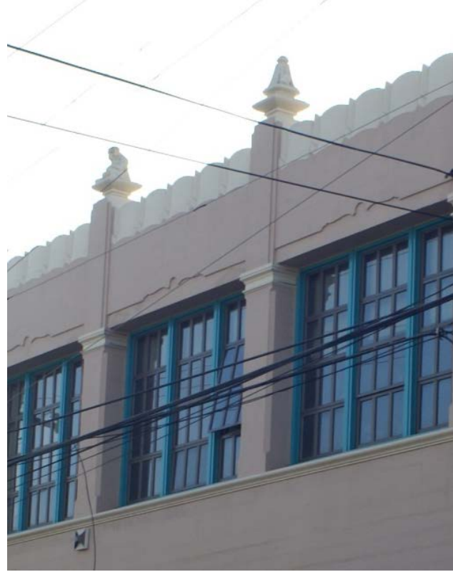
Figure 19. Typical condition at second floor level of east classroom wing facing Bryant Street.
