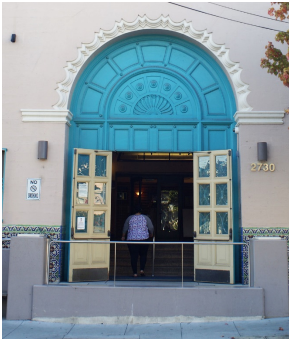
Figure 16. Detail of Bryant Street entrance.
