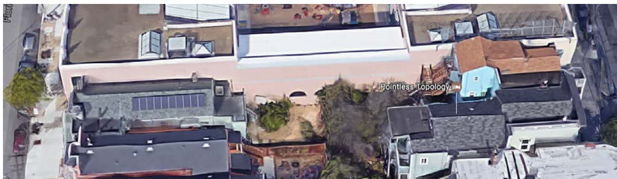
Figure 25. South façade of the Sunshine/Hilltop School; view toward north. Source: Google Maps
