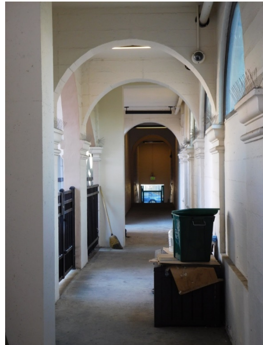
Figure 30. Passage at first floor level; view toward east.
