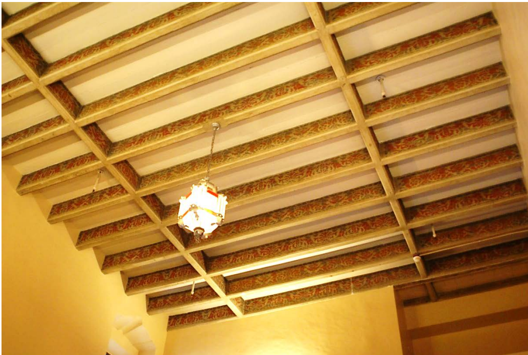
Figure 35. Ceiling of main lobby/stair; view toward north.
