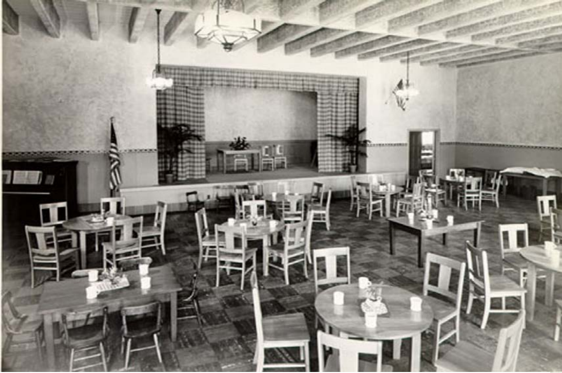
Figure 54. Dining room on second floor of the Sunshine School, 1937.
