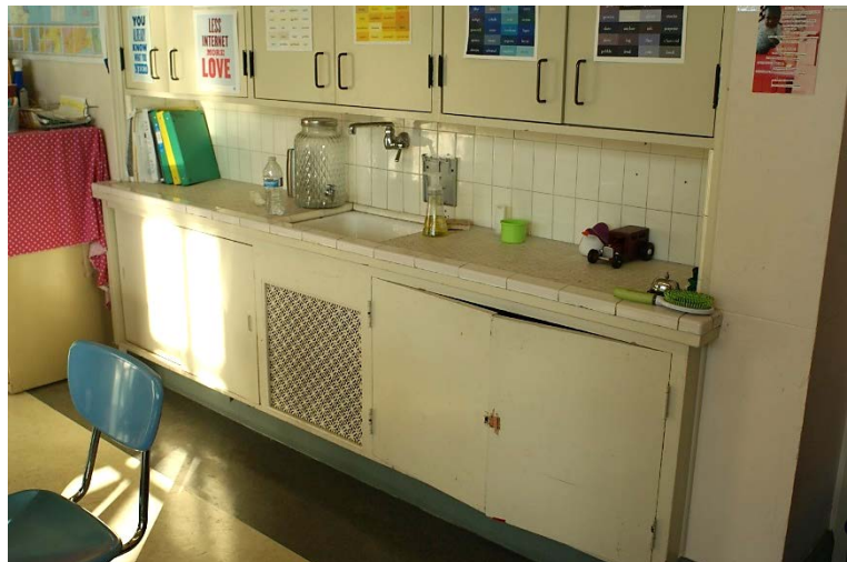
Figure 42. Sink and cabinets in a typical classroom.
