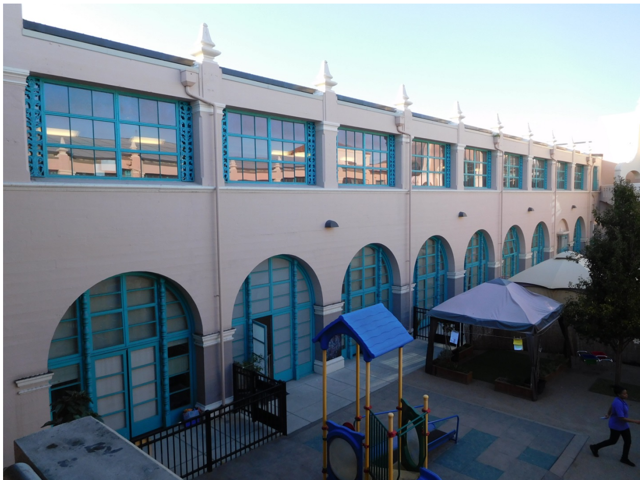
Figure 28. West side of the courtyard of the former Sunshine School; view toward northwest.
