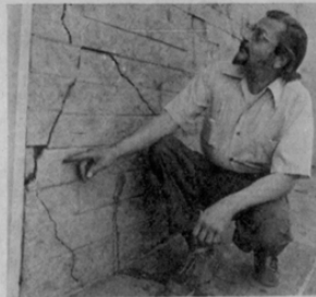
CUSTODIAN JOHN CASE CHECKS CRACKS IN WALL. Structure is moving sideways and down at some time.
