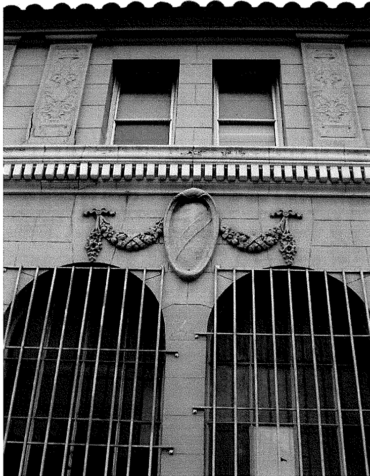
3. Detail, southern end bay of front facade, 650 Divisadero Street.
