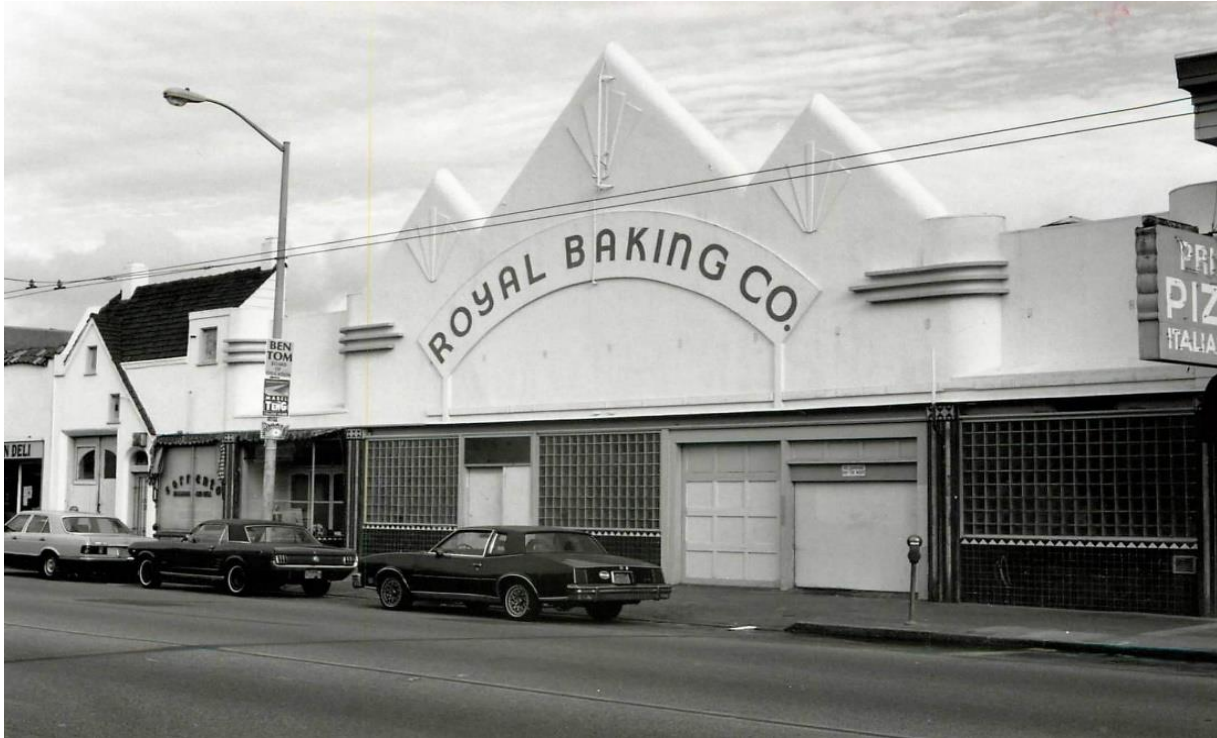
4769-4773 Mission Street, November 1990. Source: San Francisco Heritage.
