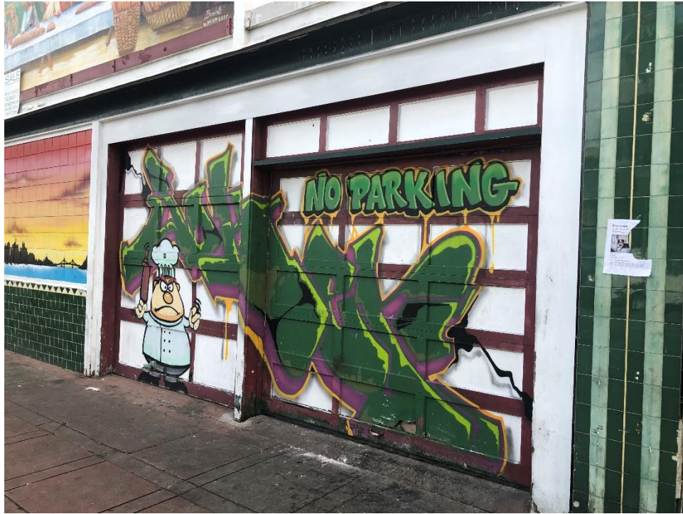
Original garage bay openings with replacement garage doors at 4773 Mission Street, January 2020.
