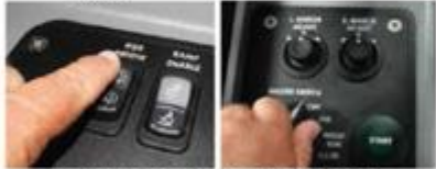
Figure 21-12. Maximize Ride Height and Turn OFF Master Switch
