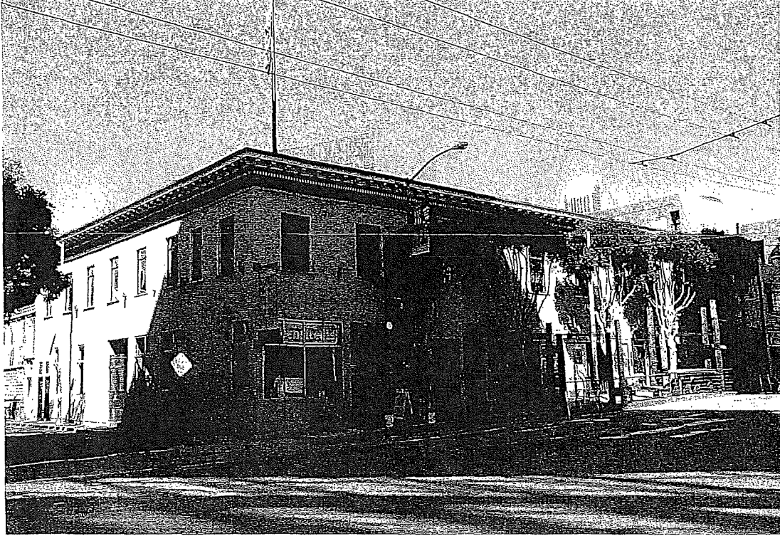
228-248 TOWNSEND STREET NEW PULLMAN HOTEL
