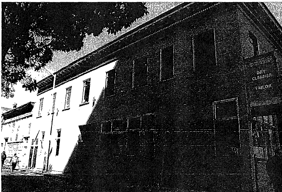
Secondary elevation (Lust Street), view north.
