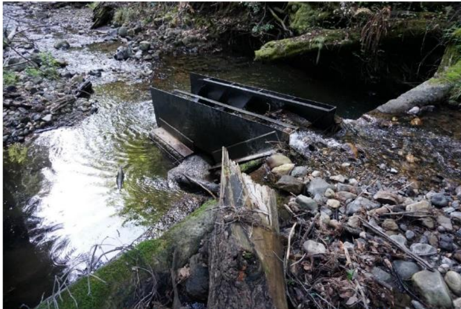
Photo 2: Dam and Denil ladder facing downstream, February 2020
