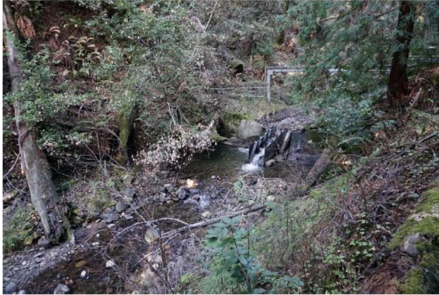
Photo 1: Dam and Denil ladder facing upstream, February 2020
