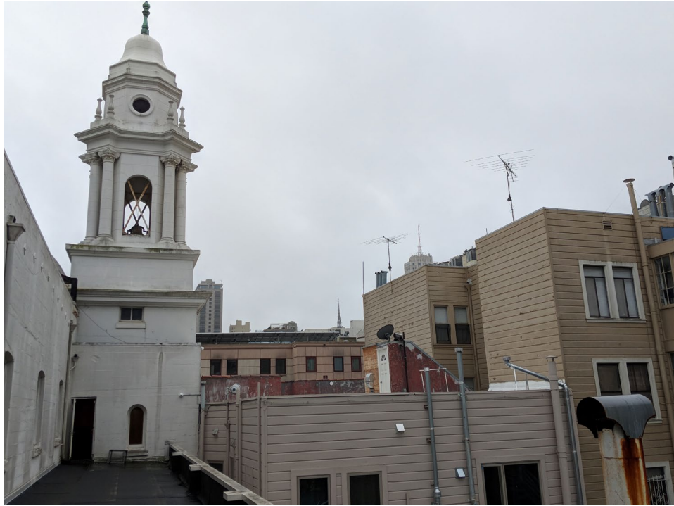
Twin tower on western portion of building exterior, view south.
