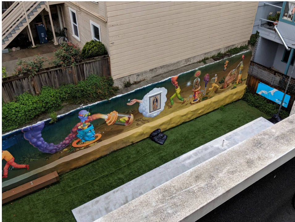
View of rear side yard from roof, view northeast.
