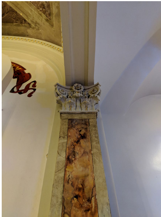
Detail of Corinthian pilaster.
