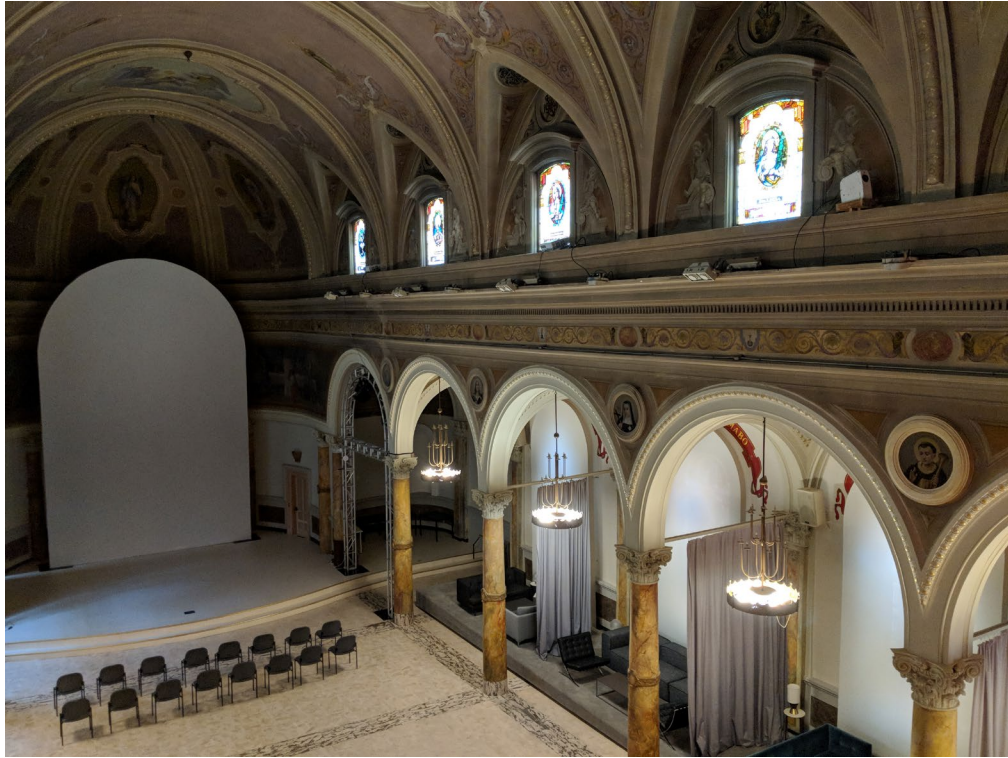
View of sanctuary from organ loft, view northeast.
