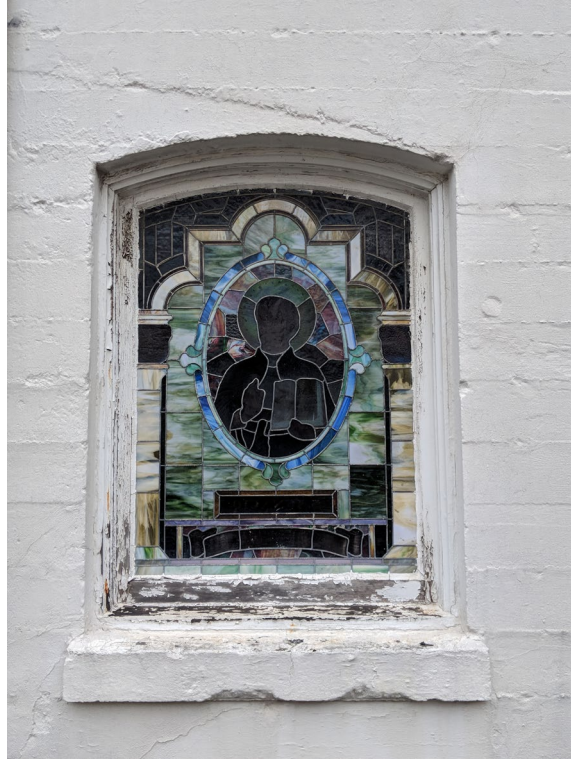
Exterior view of clerestory stained glass window, view east.
