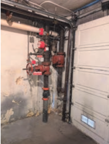
GROUND FLOOR - FIRE WATER ASSEMBLY
