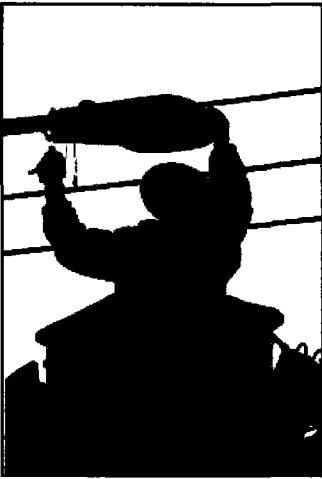
LED Streetlight Installation
