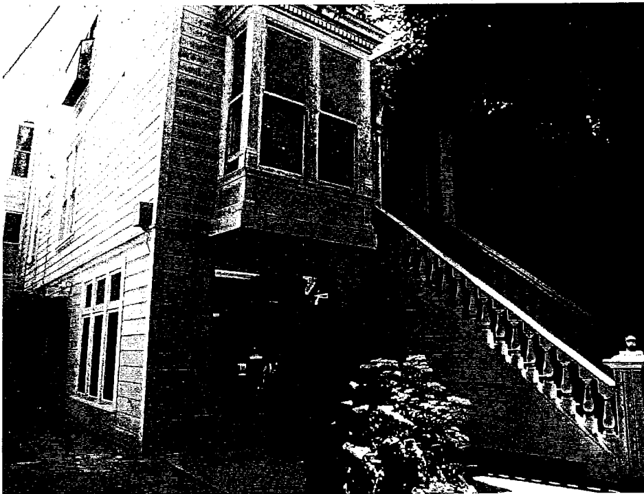
Figure 1: 1712-1716 Fillmore Street, view looking southeast.
