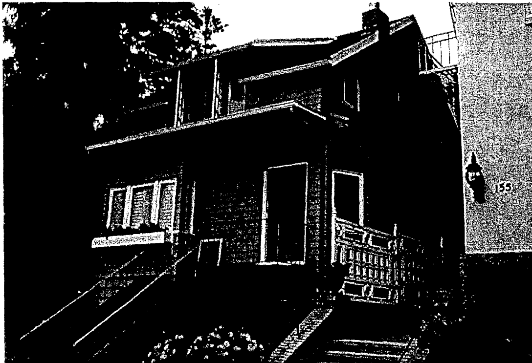
LOOKING SOUTHWEST FROM 24 TH AVE. TOWARDS 157 – 24 TH & CATCHING 155-24 TH
