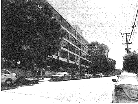
6th Ave between Geary and Anza (Kaiser medical Building. Verizon)
