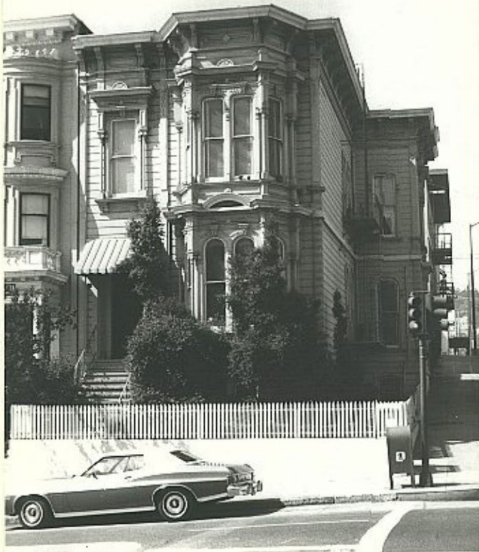
Source: DCP 1976 Survey
