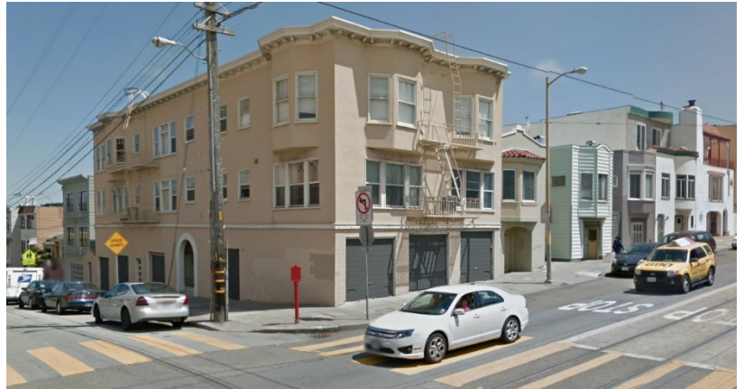
A 6-unit building adjacent to a 3-unit building (left) and a single-family home (right) in an RH-2 District in the Inner Sunset.
