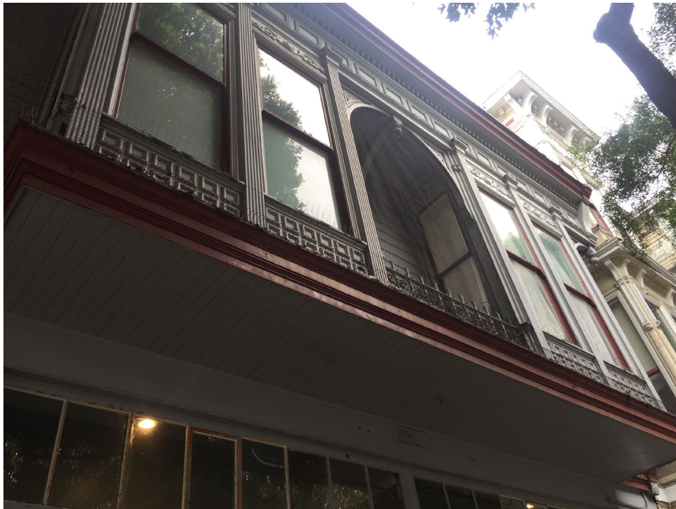
Upper portion of 2855-2861 24 th Street, showing bay windows, view southwest, December 2018.
