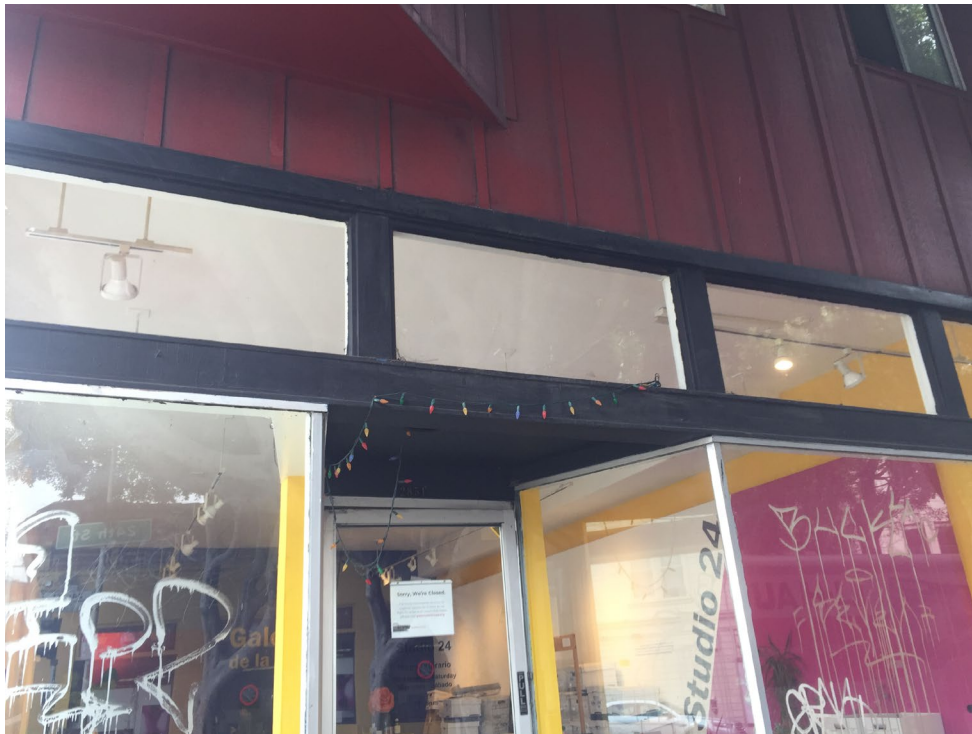
Transom above storefront entrance at 2851 24 th Street, view south, December 2018.
