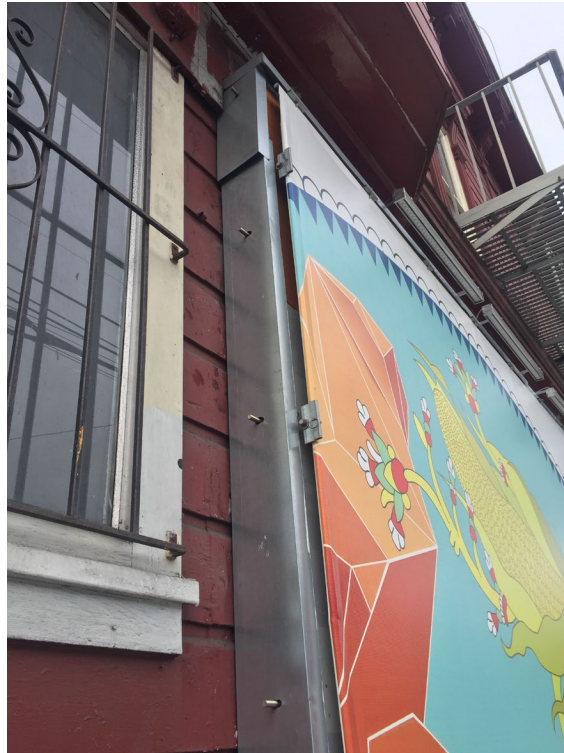
Detail of Bryant Street façade, view northwest, December 2018.
