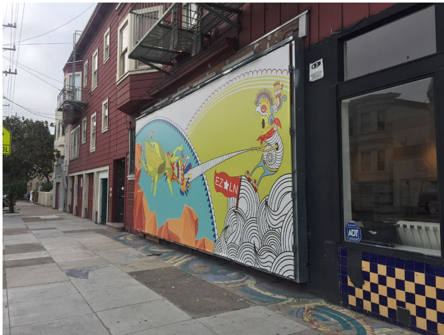
Bryant Street façade, view southwest, December 2018.
