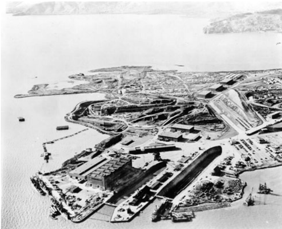
Figure 1: The Shipyard Under Construction
