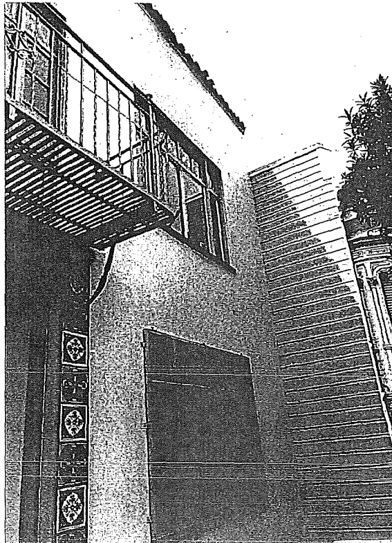
Detail at front façade, view southwest.
