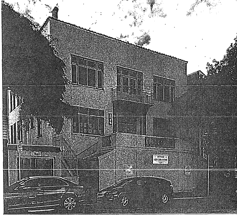
Primary elevation, view southwest.
