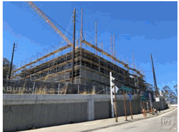
The Bristol Construction
