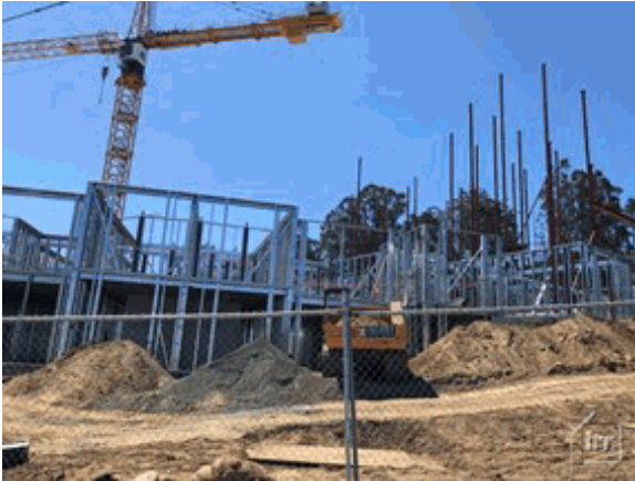
The Bristol Construction
