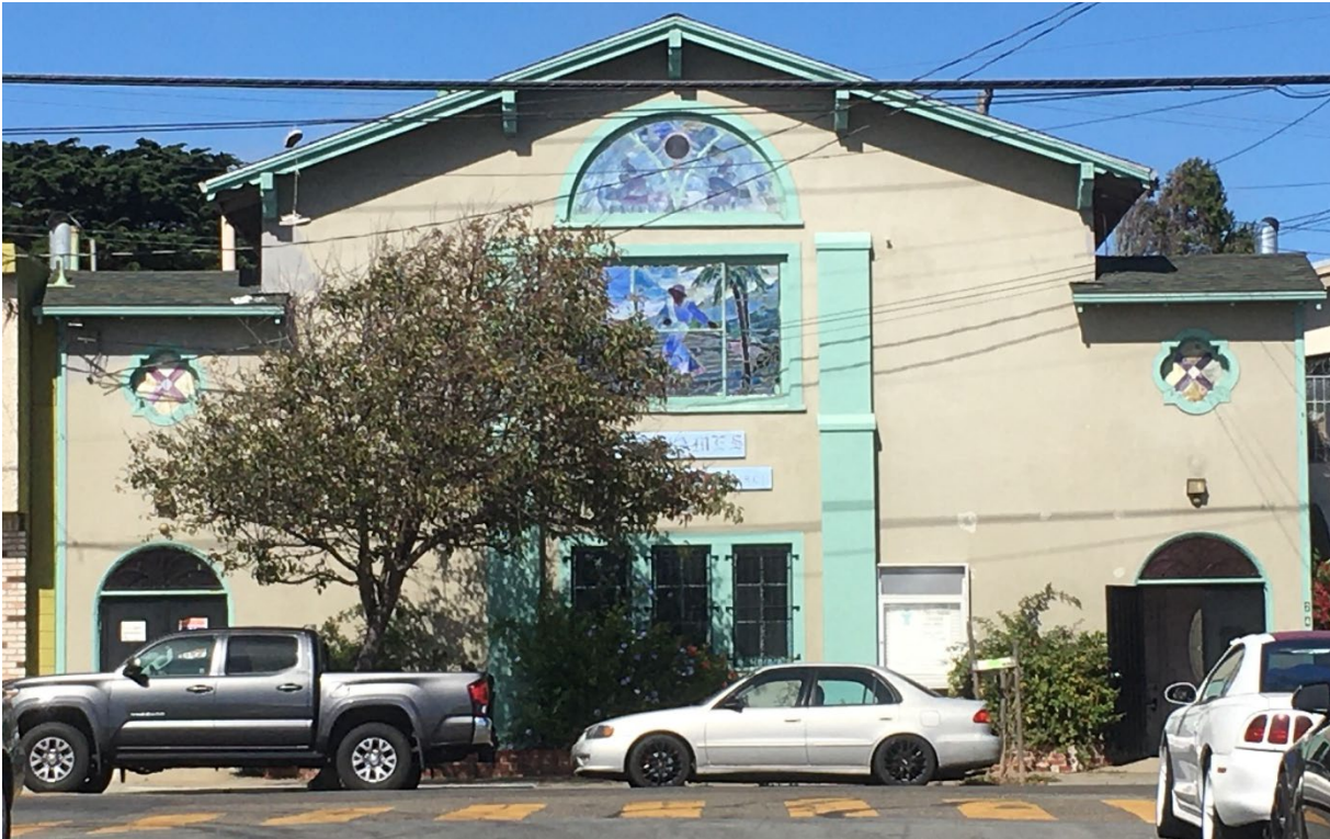
St. James Presbyterian Church, front (south) façade, view north, 2022 Source: San Francisco Planning Department
