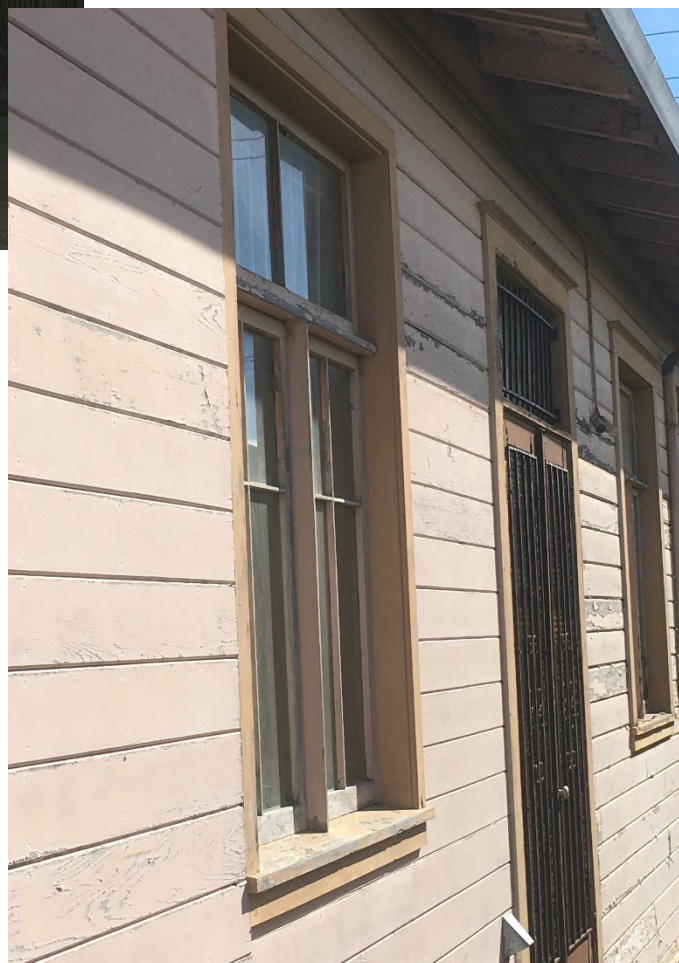
St. James Presbyterian Church, west elevation, 2022 Source: San Francisco Planning Department
