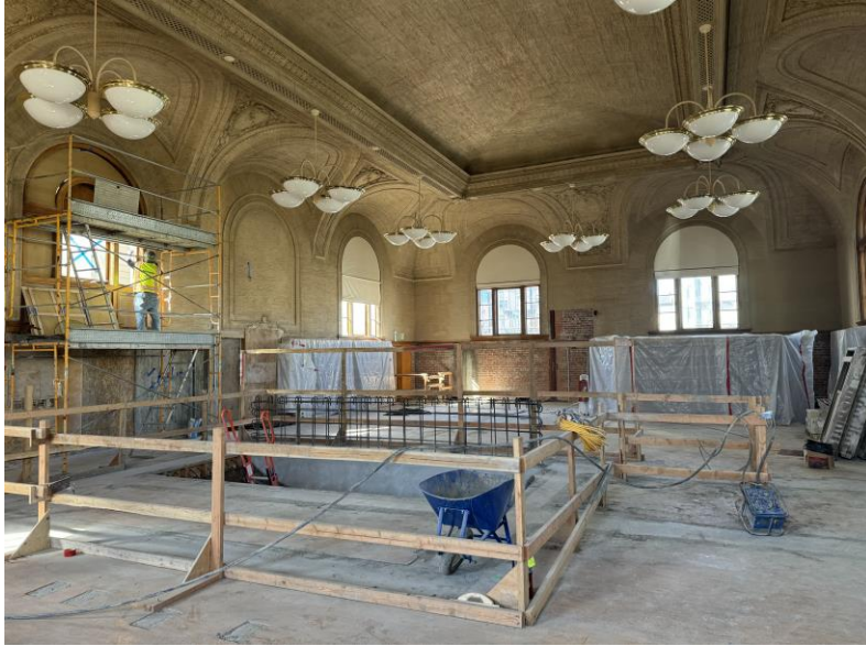
Renovation of Mission Branch Library
