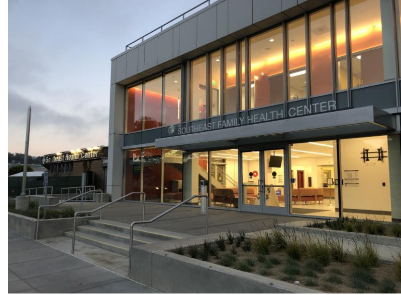
Built new Southeast Family Health Center
