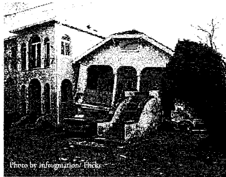
The result of a soft story collapse.
