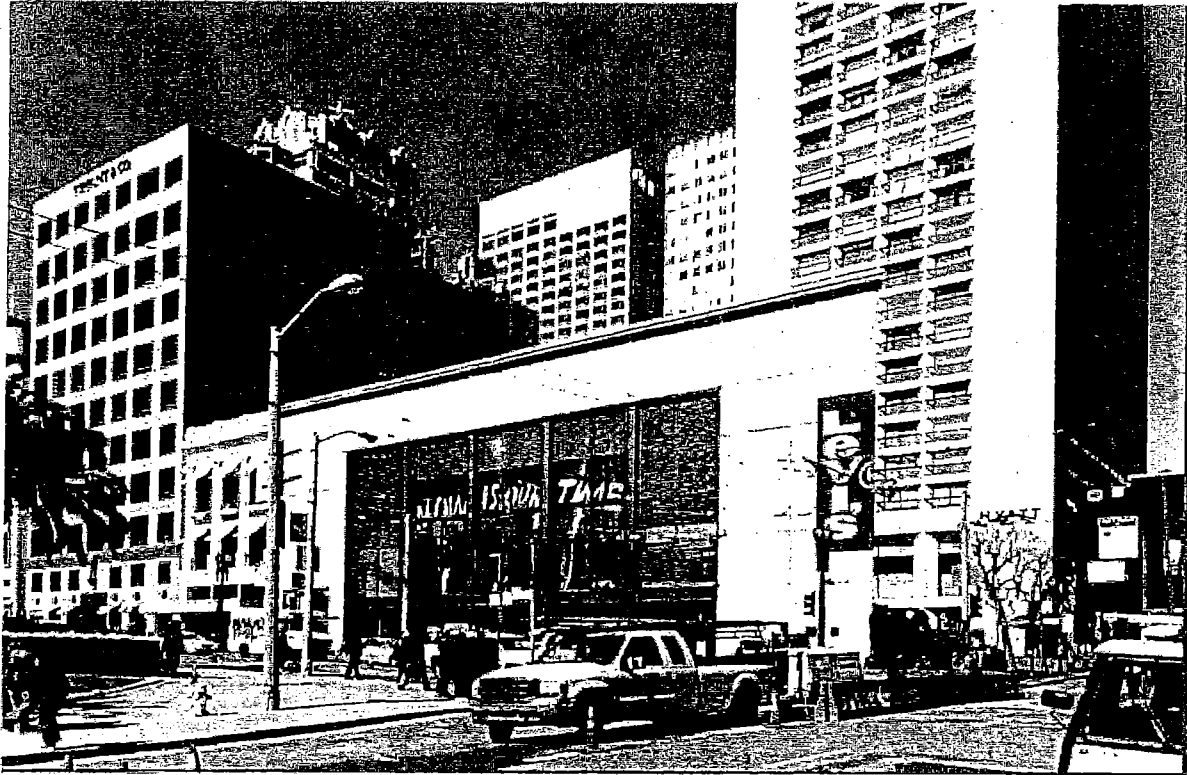
300 Post Street/345 Stockton Street
