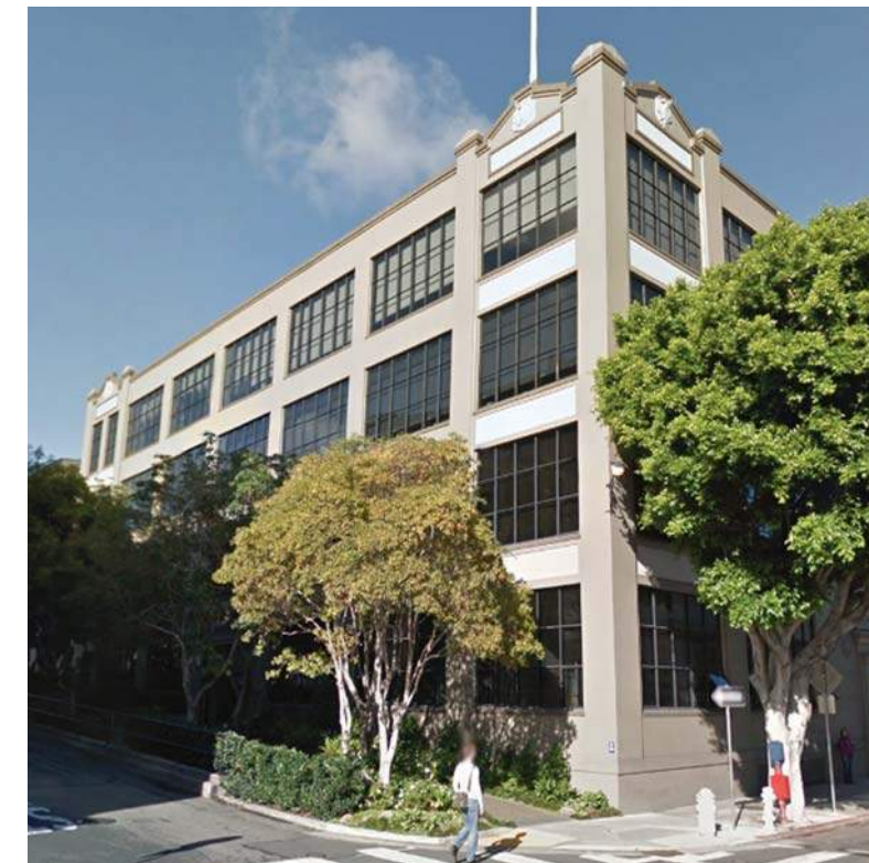
FRAME AND INFILL WITHIN DISTRICT 901 Battery St.
