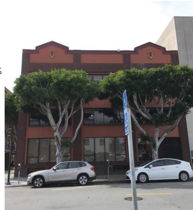
FRAME AND INFILL WITHIN DISTRICT 100-120 Broadway
