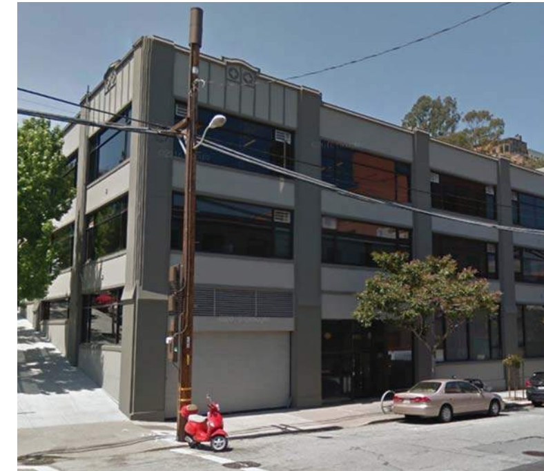
FRAME AND INFILL WITHIN DISTRICT 1005 Sansome St.
