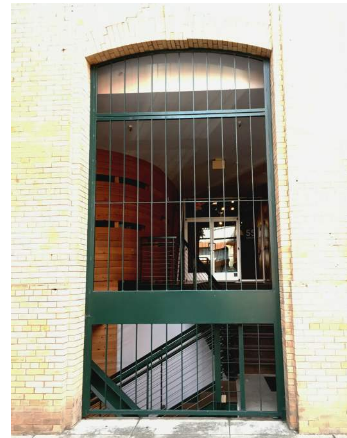
TRANSPARENCY/GATES WITHIN DISTRICT 55 Union St.
