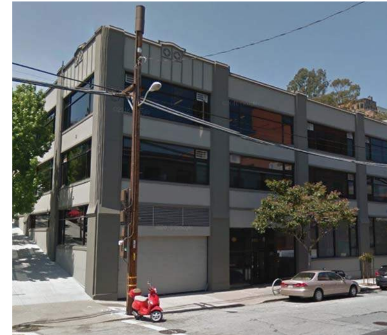
FRAME AND INFILL CORNER WITHIN DISTRICT 1005 Sansome St.
