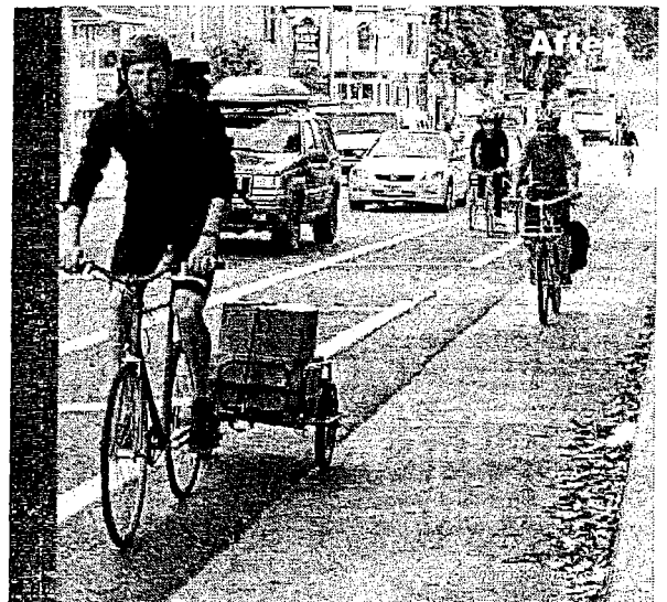
After: The SFMTA constructed the first phase of the Oak and Fell Safety Project, using buffered bicycle lanes, green pavement, and bike boxes to make this critical east-west connection a more comfortable place for people on bicycles.
