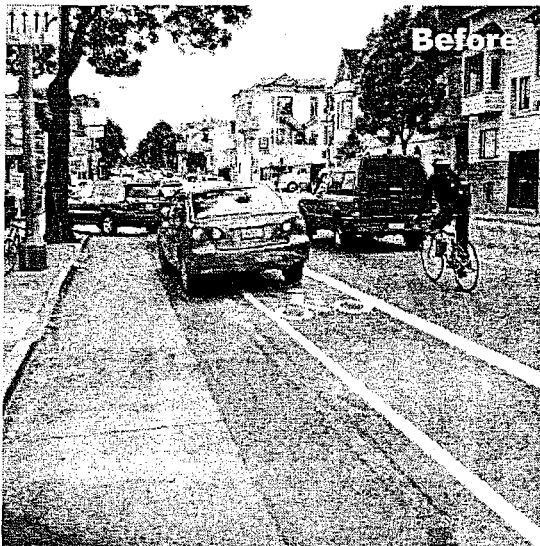
Before: The Fell Street bicycle lane between Scott and Baker had several stressful characteristics, including frequent lane blockages and proximity to high-volume, high-speed traffic.
