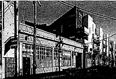
Diversity of Buildings and Architecture
