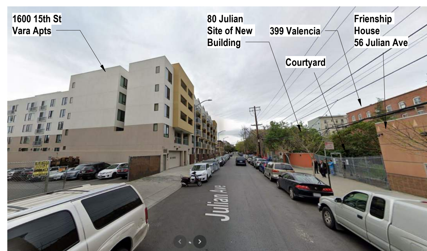
D) Julian Ave - Facing Side
