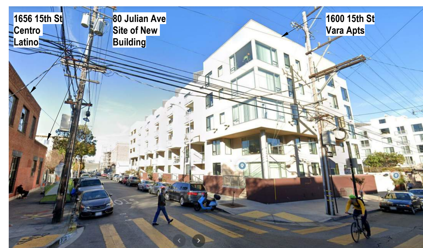
A) Julian Ave - Facing Side
