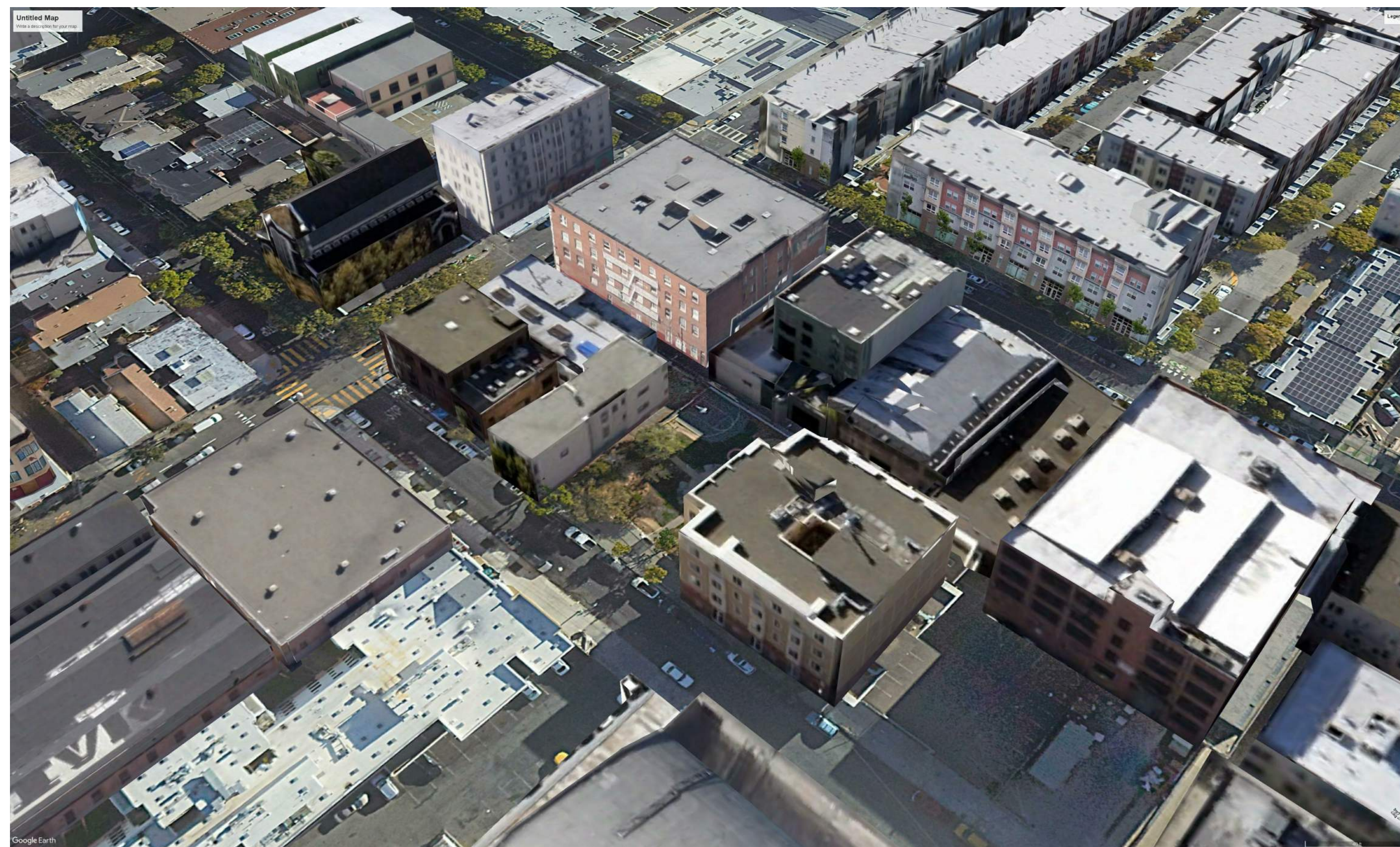
AERIAL VIEW FROM NORTH EAST - WITHOUT NEW BUILDING
