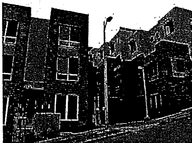
Unit pattern stepping down the street
