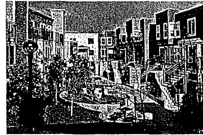
Common open space at podium level
