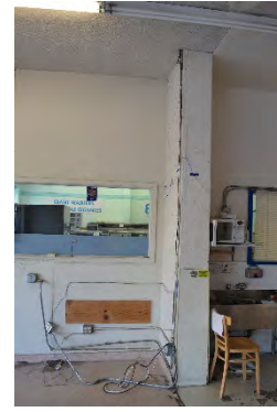
Figure 12. Two windows within the partition wall that separates laundry from vacant commercial space, facing south
