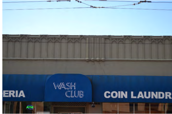
Figure 5. Gothic frieze at the parapet, east (primary) façade, facing west
