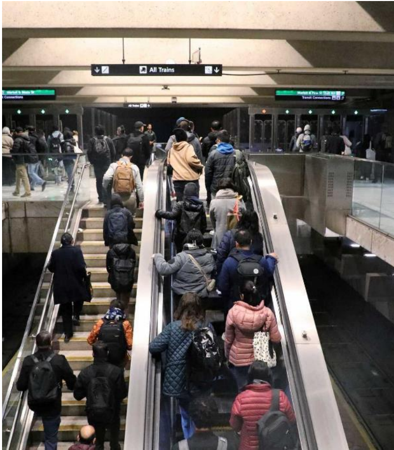
Market Street Escalator Renovation Project
