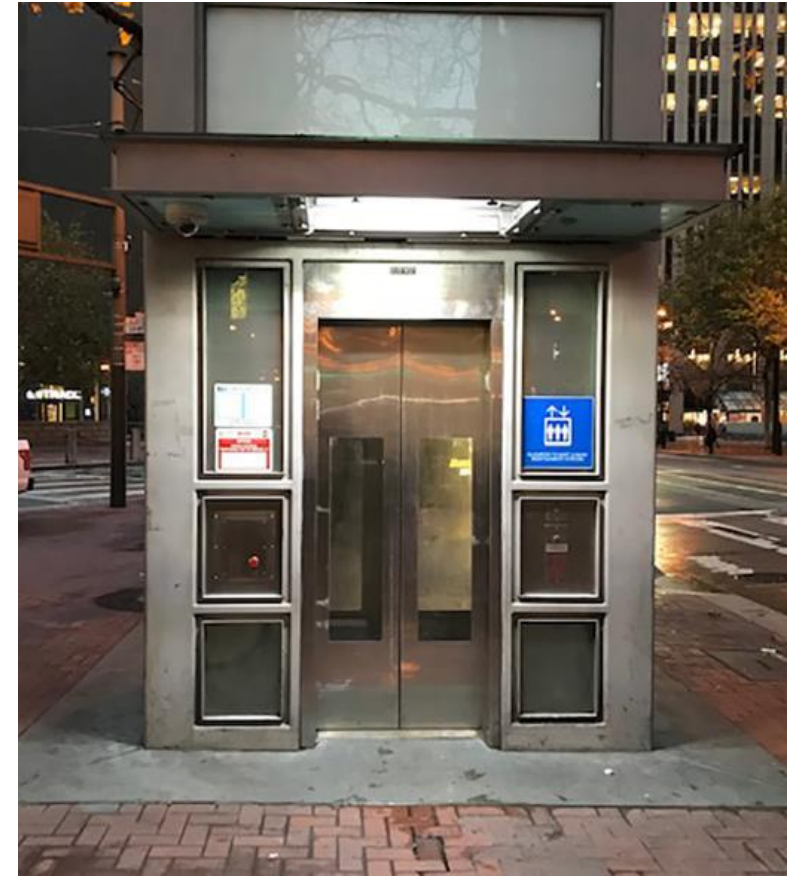
Elevator Modernization Program
