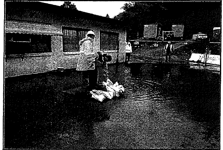
Flooding at Control Building
