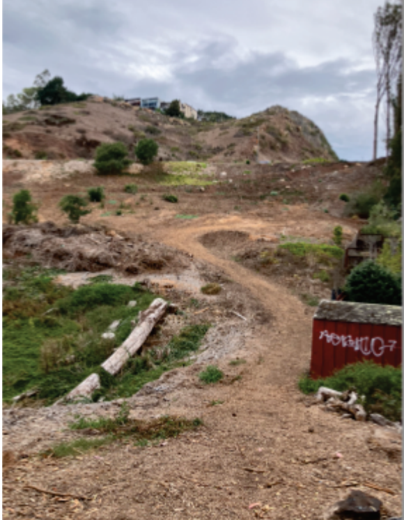
Fig. 9: PUC Tree Removal from Glen Canyon off O’Shaughnessy Blvd
