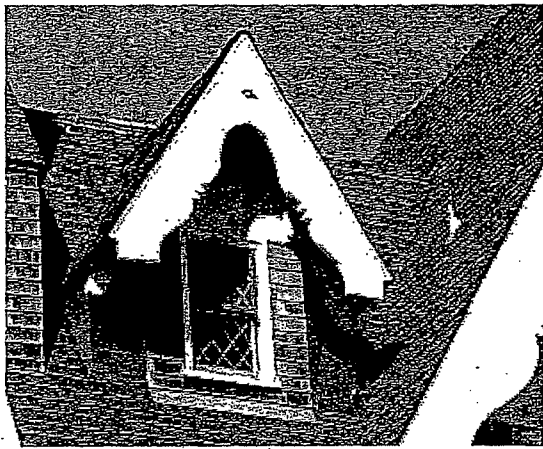
Gable dormer at the west end of the roof.
