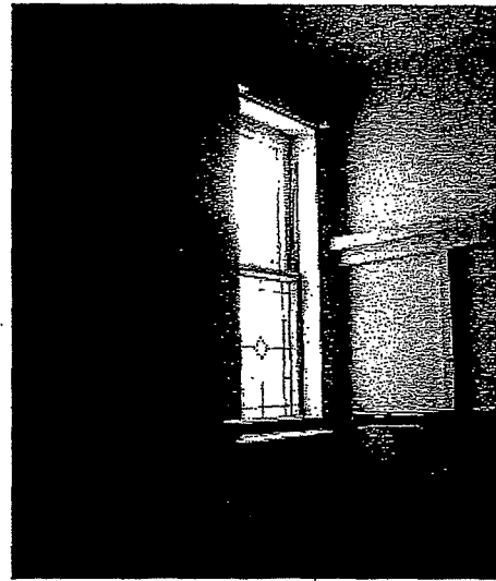
Detail of leaded glass window at the quarter-turn landing of the staircase.
