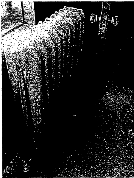
Detail of radiator in the Balder lodge room
