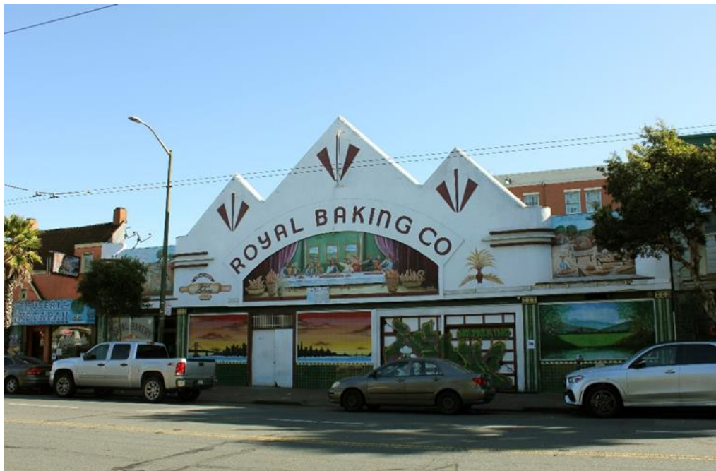
4773 Mission Street façade, January 2020.
