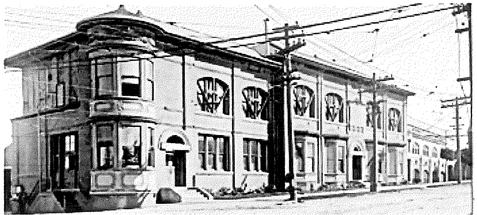
Sub-Station Building-Geneva Ave.-M.S.R.R., 1921. Courtesy of the San Francisco History Center, SF Public Library.
