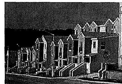
Residential units line the parking podium and
