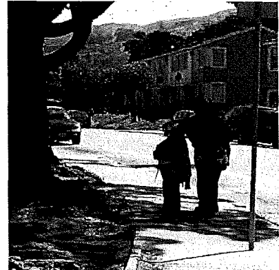
Sidewalk at Santos Street near Sunnydale. Tree roots have damaged some sidewalks in the neighborhood.
