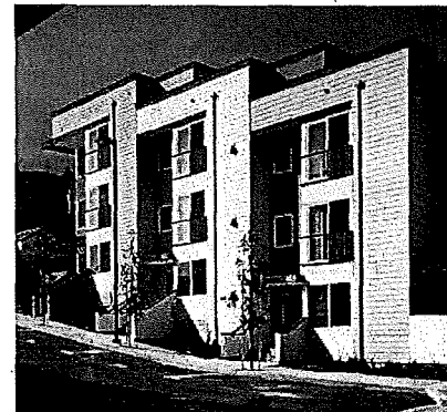
Stoop entries at ground floor units. Residential module is evident in this stacked flat building.
