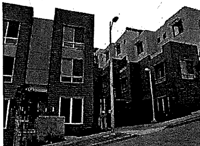
Unit pattern stepping down the street.
