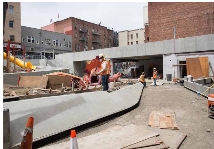
Work continues on Chinese Playground
