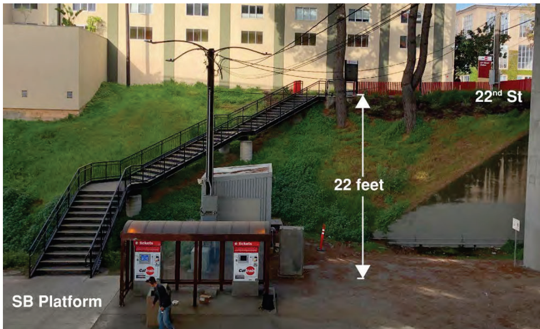
Southbound Platform Staircase
