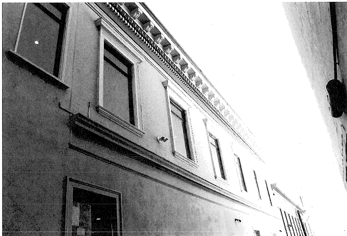
Secondary (Clyde Street) elevation, view west.
