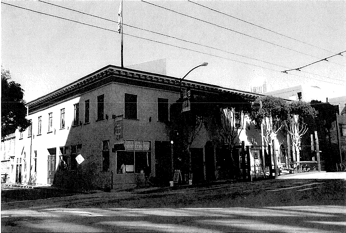
228-248 TOWNSEND STREET NEW PULLMAN HOTEL
