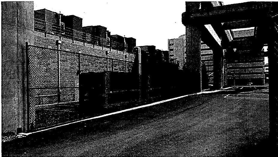
Photo 3C: Airport Data Center (Looking East)
