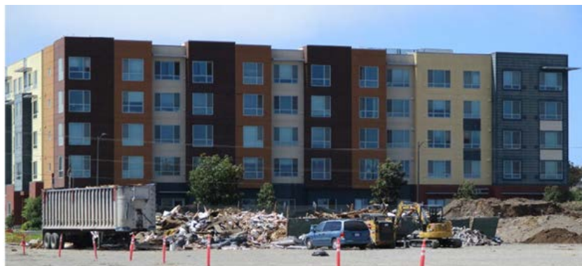
Pictured above is a recent example of illegal dumping/disposal near the Alice Griffith Apartments in the Bayview-Hunters Point neighborhood.
