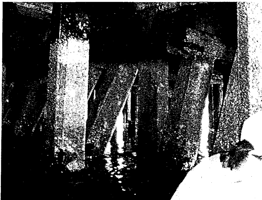
Photo 3. Typical section at batter piling along North Apron
