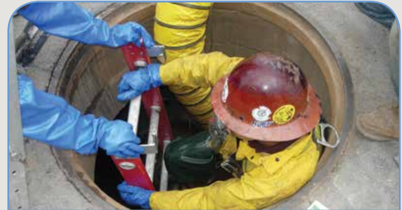
A paved working surface is needed around wastewater manholes to facilitate access to the wastewater collection system for routine inspection and maintenance.
