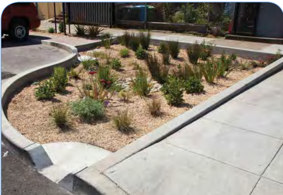
Typical Green Stormwater Infrastructure bioretention planter
