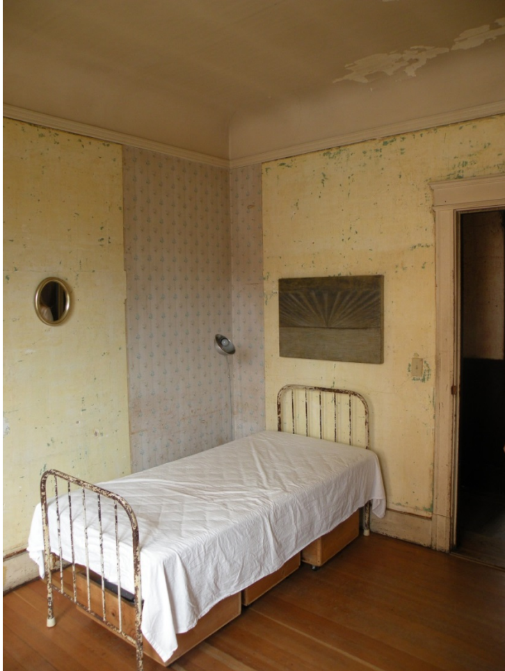
Figure 31 Early 20th Century wallpaper is retained in a portion of this bedroom at 194 Gough Street and is the first wall treatment over the lathe and plaster. Note the original surrounds, hardwood floor, and cove ceiling.
