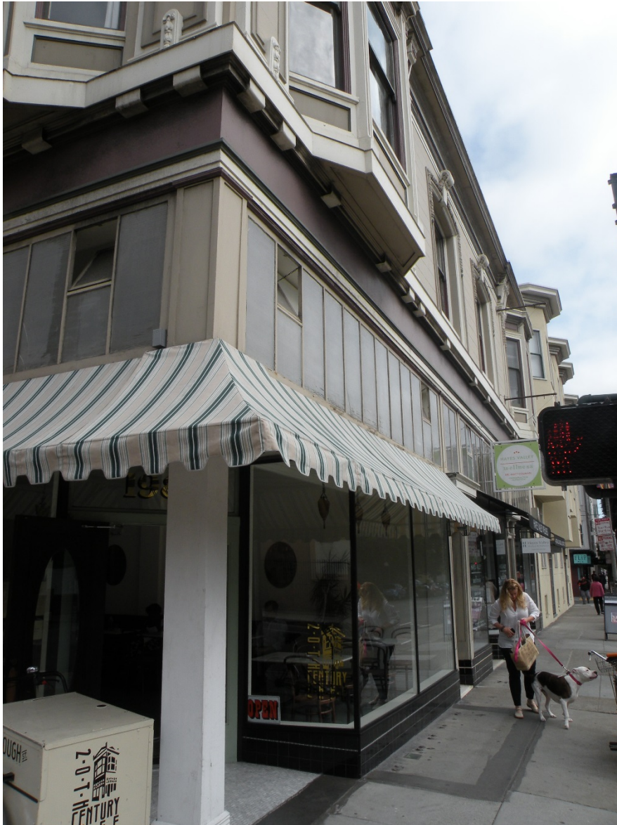
Figure 10 The commercial facade of 198 Gough St. viewed to the south.
