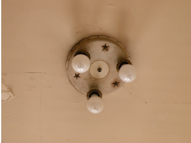
Figure 33 An original ceiling light fixture in a bedroom at 194 Gough Street.
