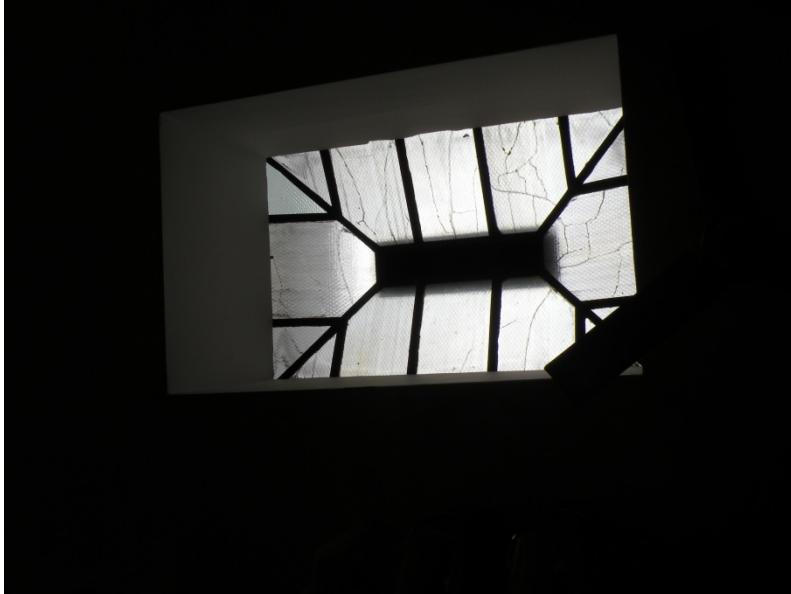
Figure 43 Looking up at the hip-form skylight in the center of the ceiling of 190 Gough Street. The skylight is set at the foot of the central light well.
