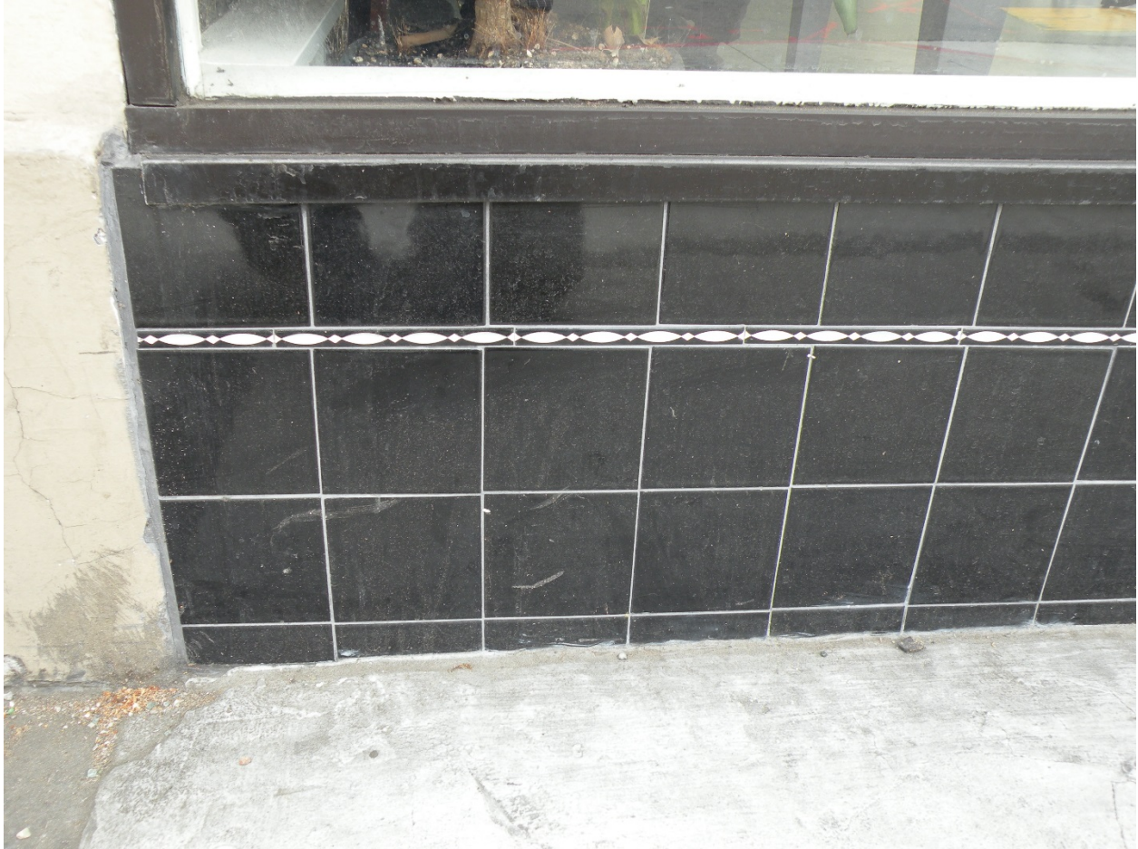
Figure 5 Black tile bulkhead with lozenge and bead narrow course as seen here at the east end of 198 Gough Street's commercial facade on Oak Street.
