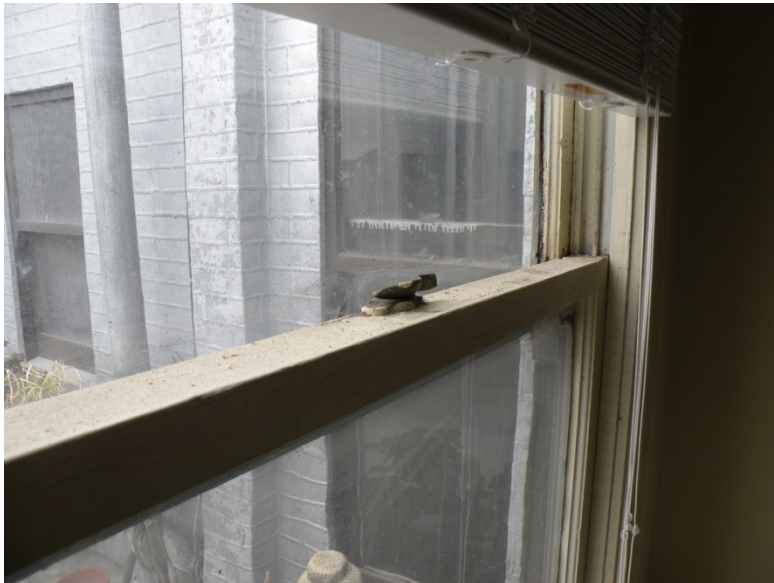
Figure 23 The large, central light well, note pressed tin cladding on the interior is impressed as faux bricks.
