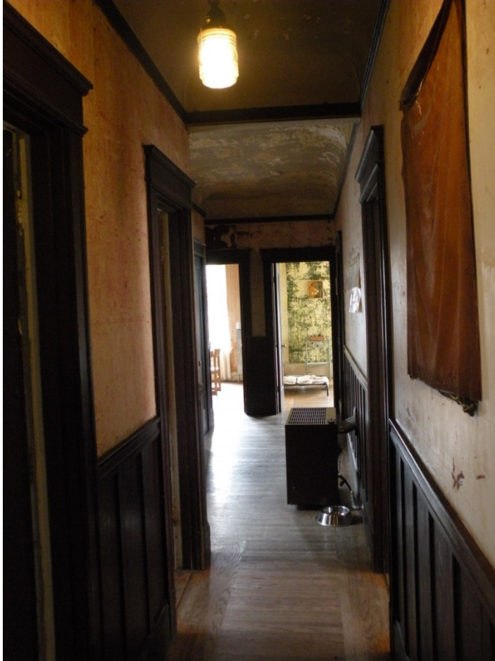
Figure 26 A view down the hallway of Rube Goldberg's apartment shows original finish on the woodwork including wainscoting, surrounds, picture rails, and floor. The hallway, like the rooms off of it, has high cove ceilings. A second gas heater from the third quarter of the 20th Century is set in the hallway.
