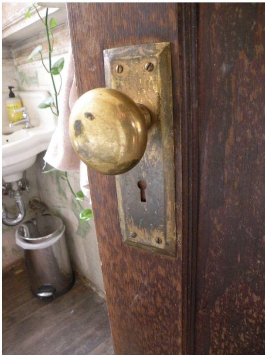
Figure 34 Hardware of brass and bronze from 1911 remain in the residential and much of the commercial units of the building.
