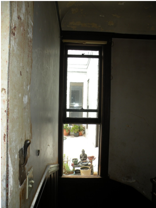
Figure 28 A view from the landing above the stairwell leading down to the front entrance at 194 Gough Street. Note the bright interior of the silver-roof light well.
