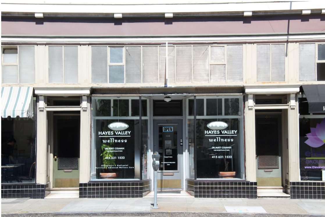
Figure 8 The commercial facade of 188 Gough Street flanked by the residential entrances to 194 Gough St. (left, Rube Goldberg's residence) and 186 Gough St. (right, Max Goldberg's residence).
