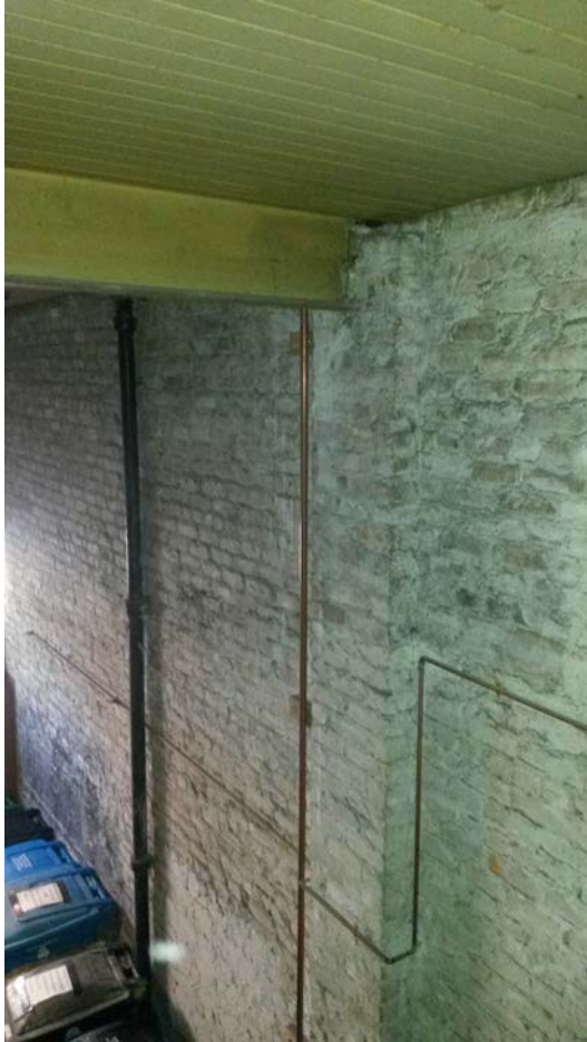
Figure 15 Steel frame visible at the utility area at the east end of the building. Note the I-beam and brick-veneer pilaster containing the steel column at the intersection of the northern and central structural bays. View of the east wall, photographed to the northeast.
