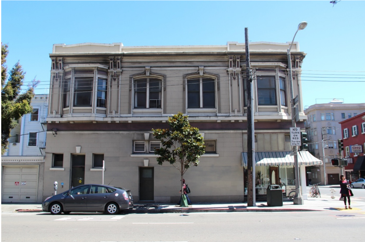
Figure 18 View of the Oak Street elevation, the entirety of the second floor that is visible here was the residence of Rube Goldberg. The north-facing elevation is replete with windows and northern light, a perfect work environment for the visual artist.
