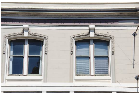
R. L. Goldberg Building, 182-198 Gough Street
