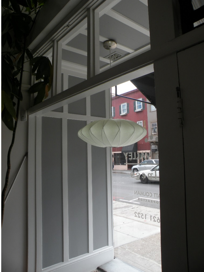
Figure 9 The tripartite transom windows and wood paneling of the 188 Gough Street. This finished carpentry remains in all the display windows of the three commercial spaces.
