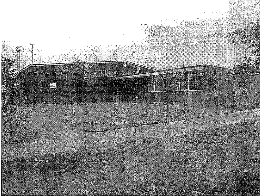
West Elevation of the Marina Branch Library.
