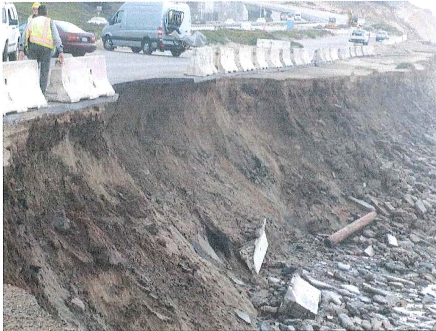
Figure 2. Eroding shoreline and rubble at South Ocean Beach, February 2016.
